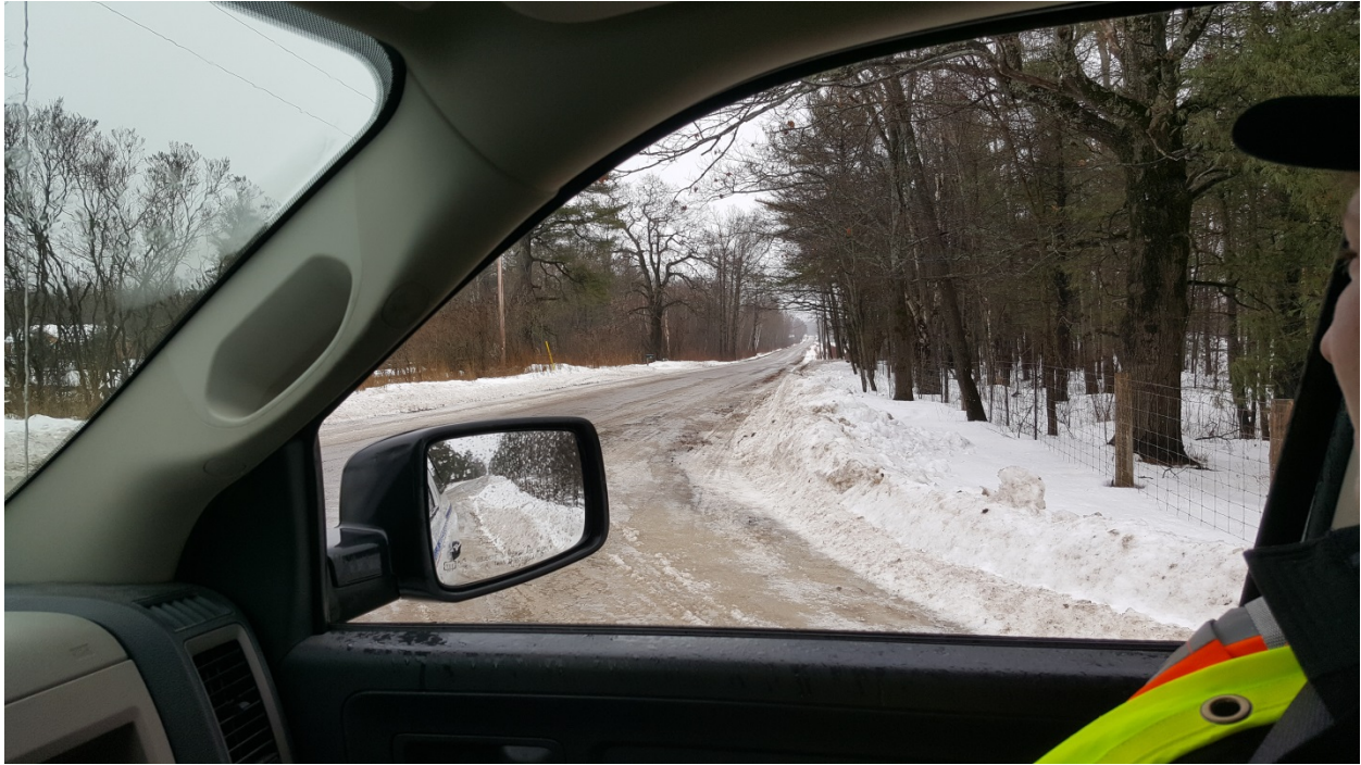
At Farmer's Rd approach T-stop control checking south sight lines
