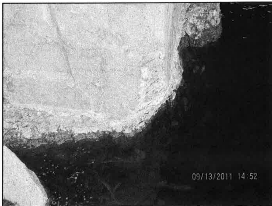
Photo 4: Severe erosion of north abutment footing
