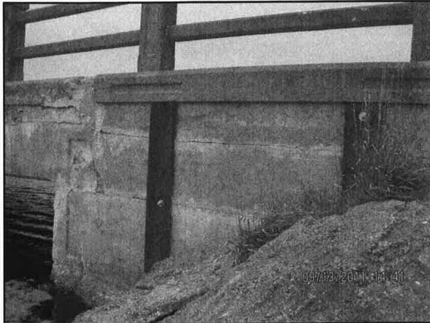
Photo 3: Wide cracks and spalls on northeast wingwall
