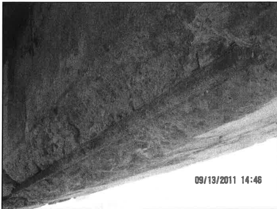
Photo 6: Spall and delamination on exterior west beam
