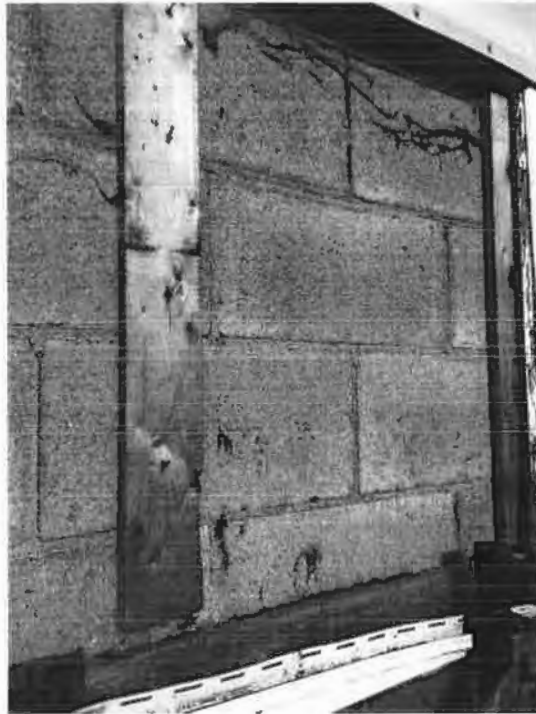
Photo #1 – Exposed 10" block above window
