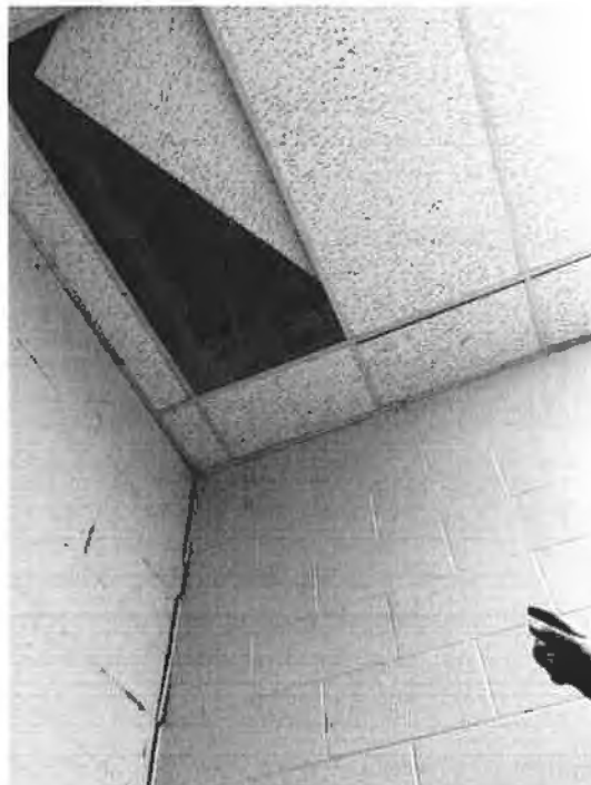
Photo #8 – Gap between interior partition wall and exterior south wall
