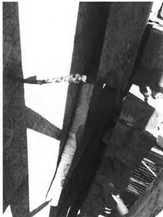
Photo #3 – Portion of brick tie perpendicular to the wall
