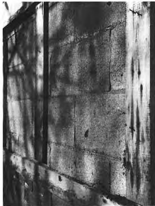
Photo #4 – Cracks at 10" block wall above the window
