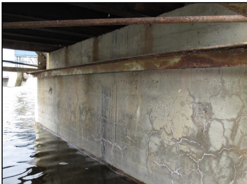
Photo 10: Map cracking at west abutment
