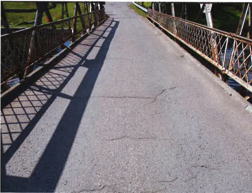
Photo 10: Medium to severe cracks at deck wearing surface
