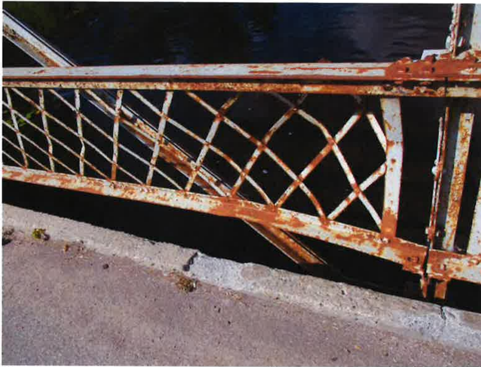
Photo 9: Impact damage at northwest
