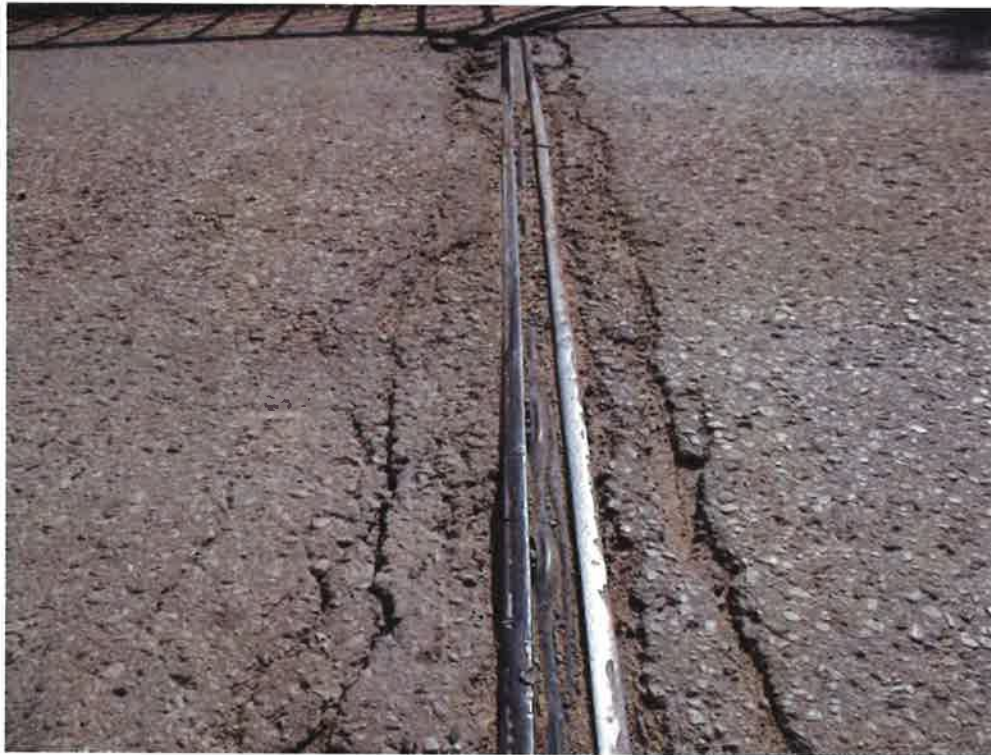
Photo 7: Severe deterioration at expansion joint assembly
