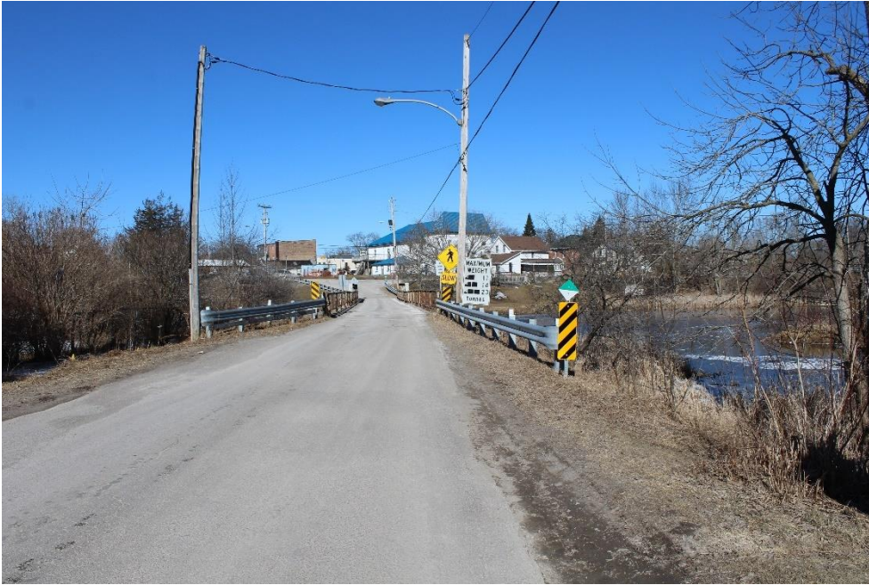
Plate 3: View of Mill Pond Bridge east approach, looking west. Note the galvanized steel flex-beam guardrails at the approaches.
