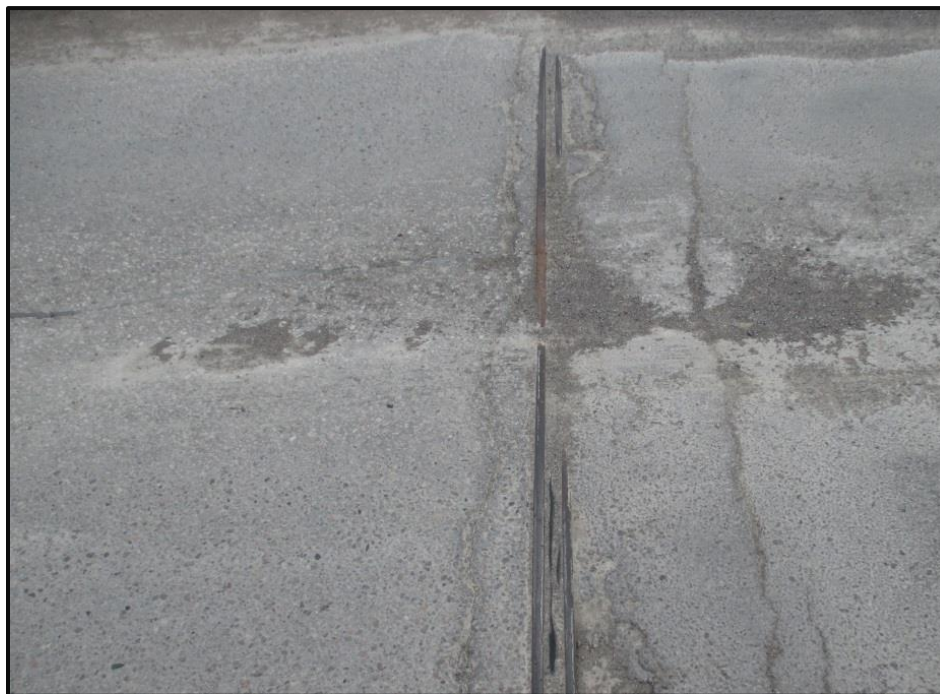
Photo 3: Jammed joints (typical of both ends)
