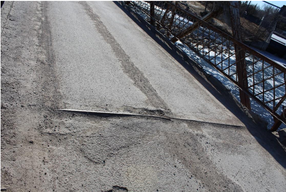
Plate 12: Detail of the western steel expansion joint on the bridge.
