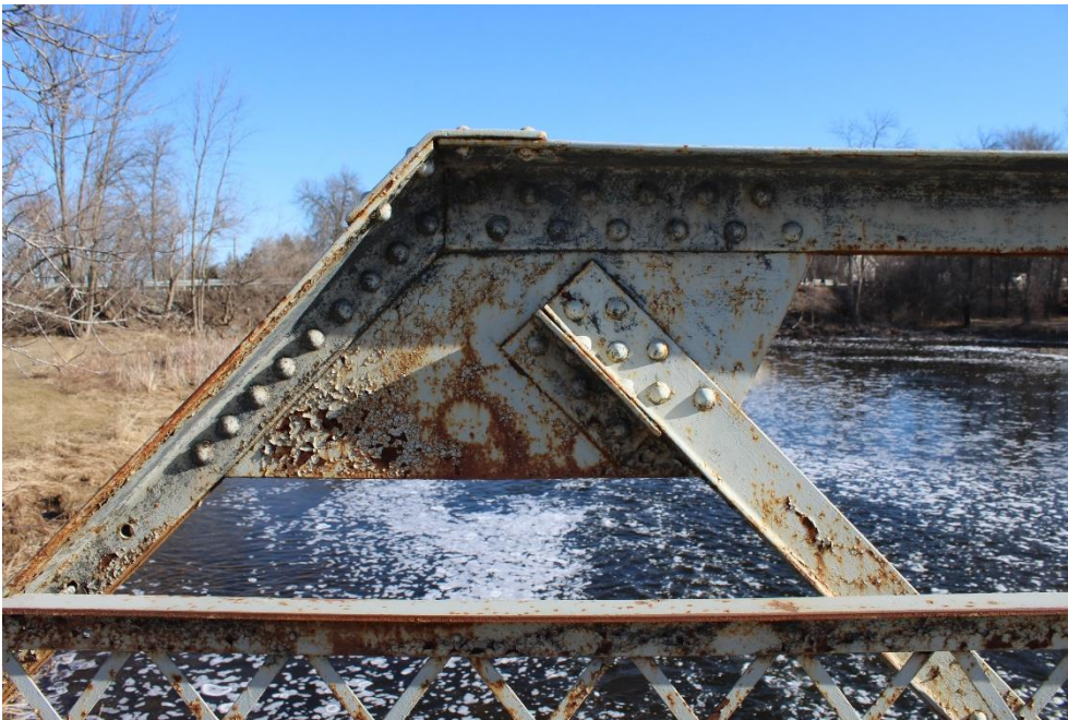
Plate 10: Riveted connection on the north portion of the west portal of the truss.
