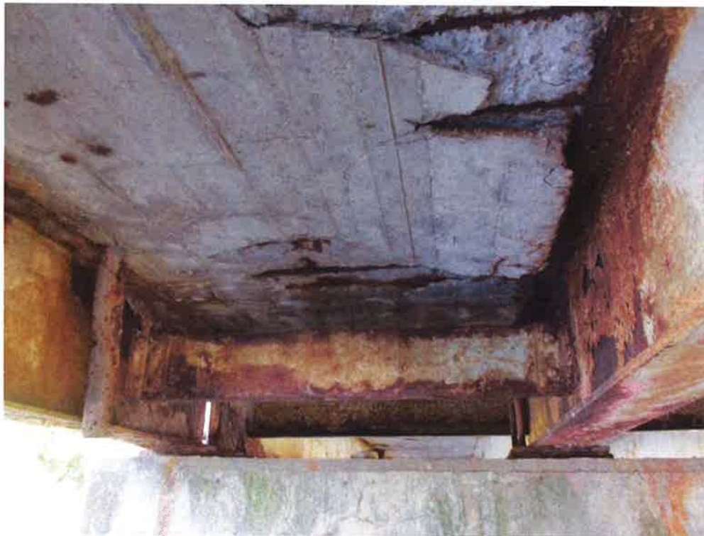
Photo 14: Severe spalls and delaminations at soffit interior
