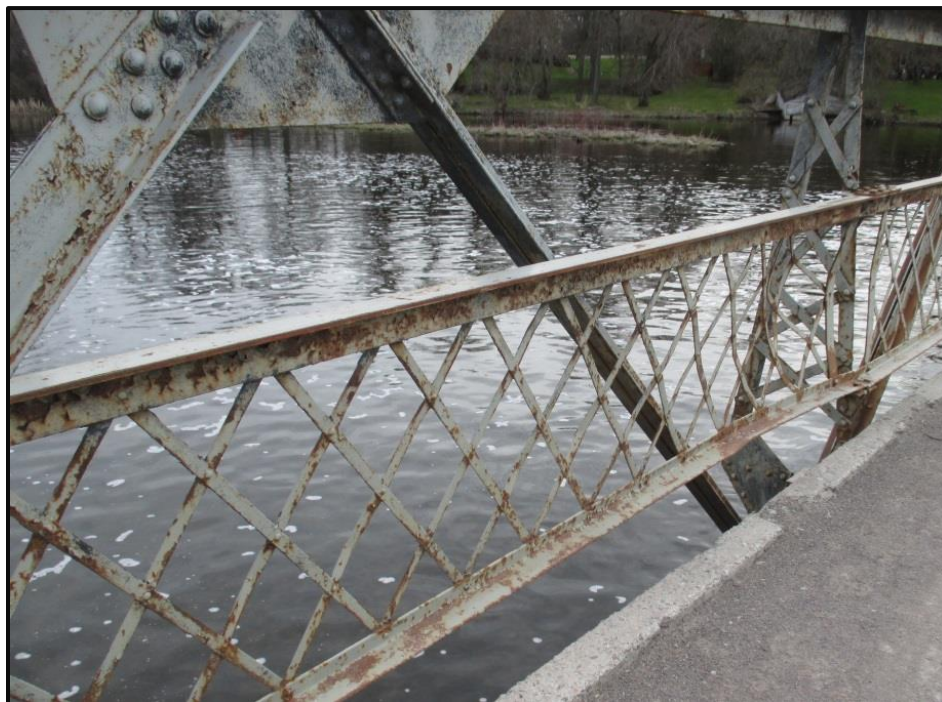
Photo 5: Deformed railing
