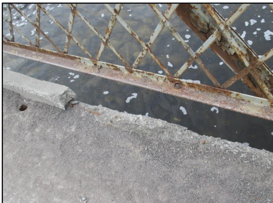
Photo 4: Typical spalling at curb
