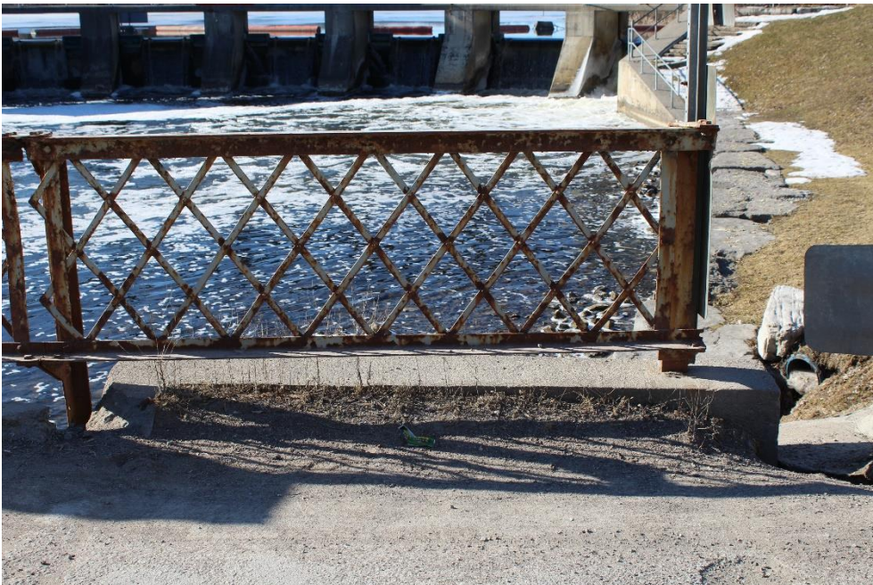
Plate 8: General corrosion along the barrier steel lattice barrier on the southwest portion of the structure.
