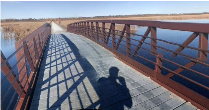
Figure 19: Ken Reid Park Bridge (VRT 008) in Kenrei Park, half-through truss, constructed in 2000. Source: Courtesy of Google Streetview
