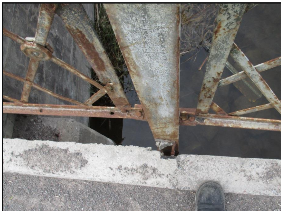
Photo 6: Broken post at southeast
