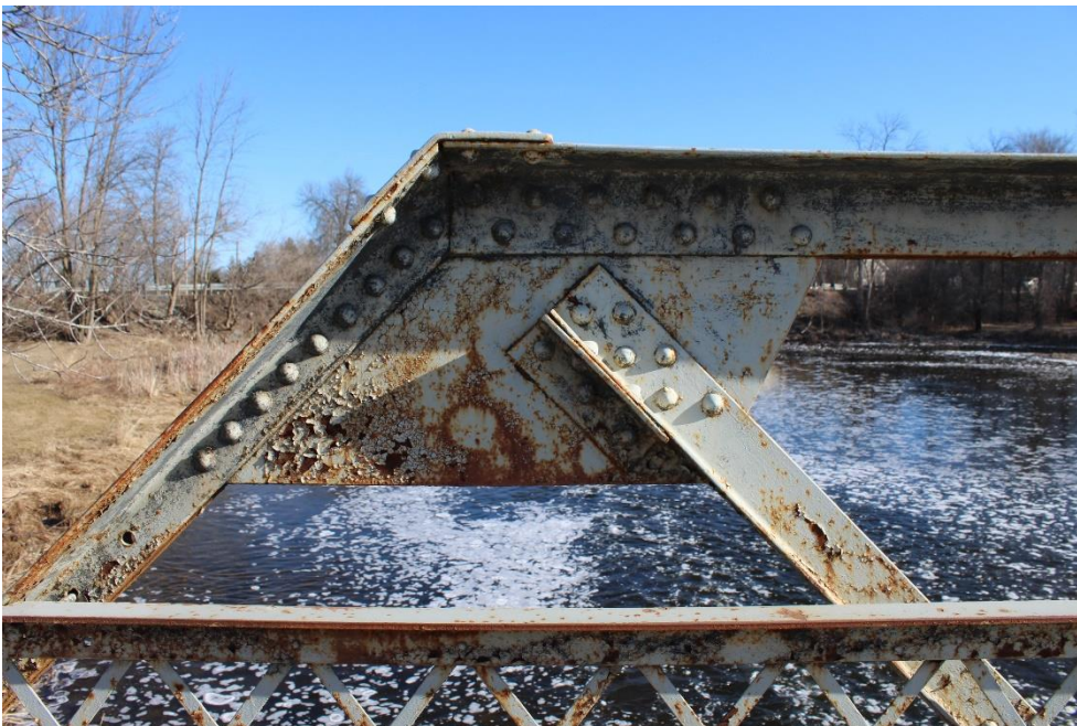
Plate 20: Riveted connection on the north portion of the west portal of the truss.
