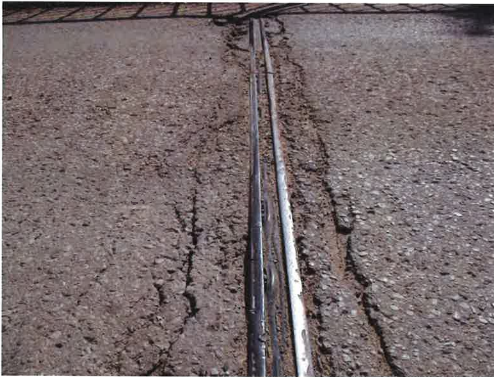
Photo 7: Severe deterioration at expansion joint assembly
