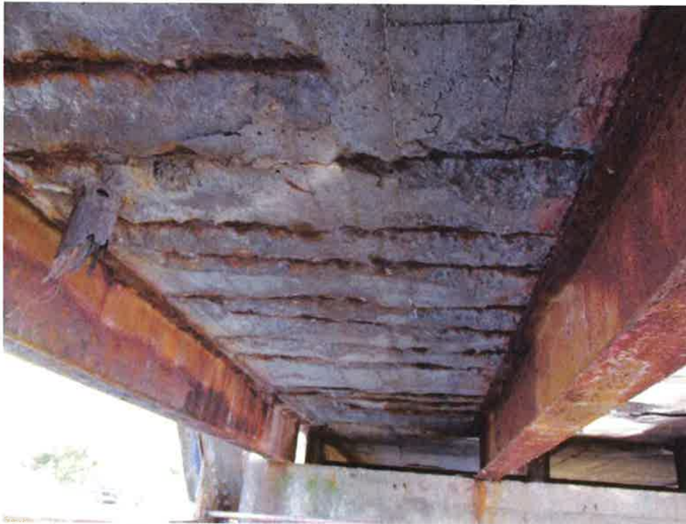
Photo 13: Severe spalls at soffit interior
