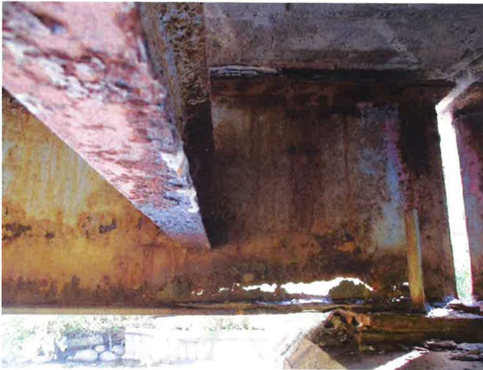
Photo 15: Severe corrosion and perforation at girder
