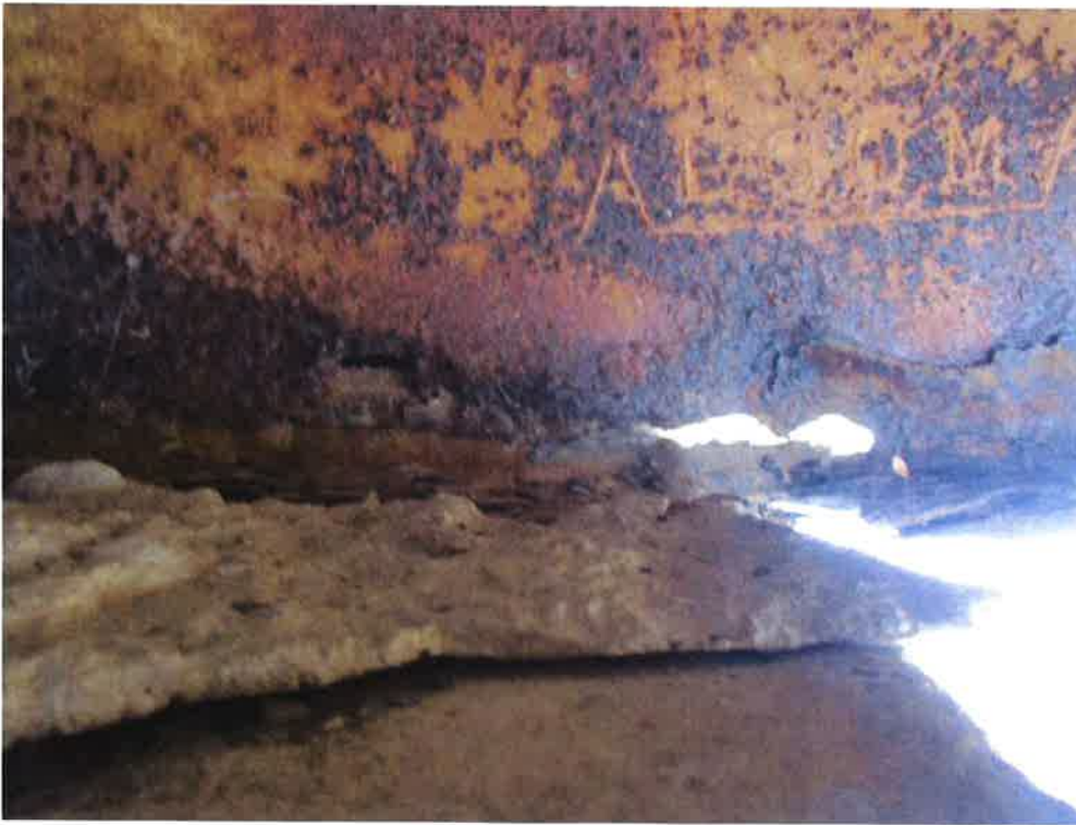
Photo 16: Severe corrosion and perforation at stringer
