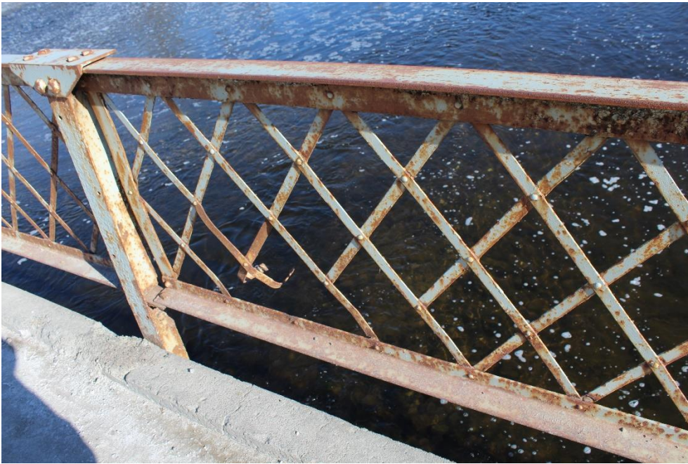
Plate 17: View of damage to steel lattice barrier.
