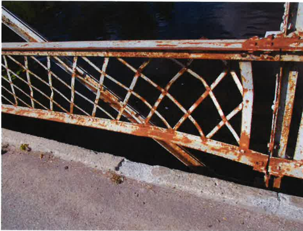
Photo 9: Impact damage at northwest
