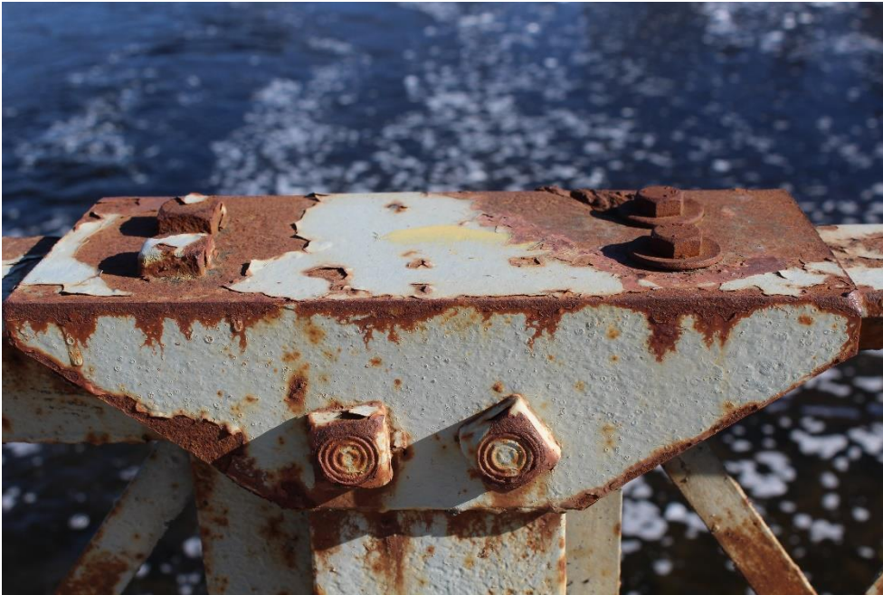
Plate 19: View of bolted joint connection along the top chord of the railing.
