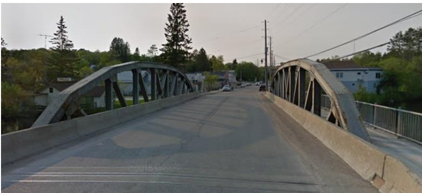
Figure 20: Burnt River Bridge (B 89406) in Kinmount, a half-through truss structure constructed in 1920. Source: Courtesy of Google Streetview
