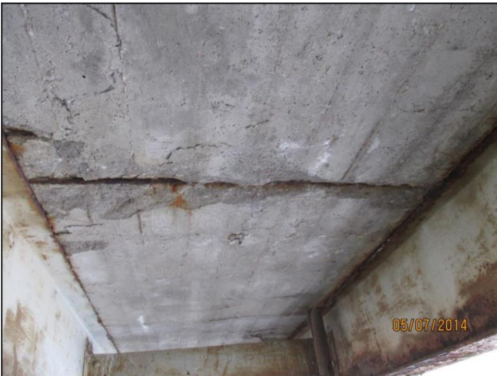
Plate 25: Concrete deterioration of the soffit of the eastern I-beam structure (DM Wills and Associates 2014).
