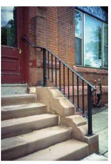
In Rehabilitation, deteriorated features should be repaired, whenever possible, and replaced when the severity of the damage makes it necessary. The stone steps of this house entrance were cracked. Appropriate work included repairing the stone steps and walls and installing a compatible metal handrail to meet building code requirements.
