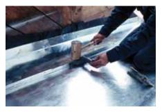
When restoring the former post office in Dawson, YK, the metal roofing surface, which was too deteriorated to repair, was replaced in kind. Physical evidence from the restoration period was used as a model to reproduce the characteristic standing seam detail.
