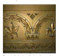
The repair of a deteriorated intricate plaster cornice should involve recognized conservation techniques, such as consolidation of the original materials in good condition. One goal should be to limit the amount of introduced material. Surface repairs may be filled with a compatible traditional plaster mix, but for larger elements, some form of adhesive or fastener may be required, and should be carefully selected.
