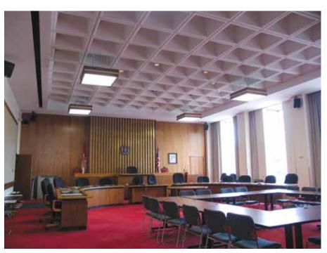
In modern buildings, reinforced concrete is often left exposed or simply painted in order to display a distinctive structural form, such as this waffle slab ceiling in the Victoria City Hall Annex. Inserting new wiring or services into such spaces can be challenging. Discreetly using conduit is recommended rather than installing false ceilings or walls that cover the historic structure.
