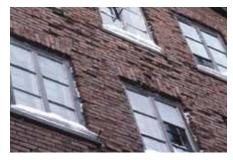
The harsh climate in many parts of Canada can seriously damage masonry elements. This wall has suffered irreversible damage from water penetrating the brick façade and freezing, causing the faces of many bricks to pop off. To avoid such damage, repair failed flashings, deteriorated mortar joints or other mechanical defects, but do not apply water-repellent coatings, which can trap moisture inside the masonry.
