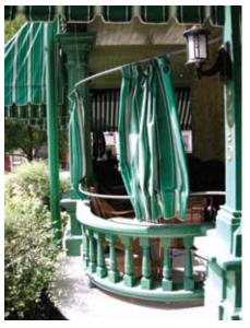
Fabric awnings are subject to damaging environmental effects including sunlight, wind and water, which eventually may cause the loss of the historic awning fabric. Repairing the original frame or mechanism and installing new awning fabric are recommended and will also help provide shade. Awning manufacturers may be able to match or provide similar fabrics compatible with the character of the place, as was done at Laurier House in Ottawa.
