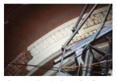
When restoring decorative plaster in the Walker Theatre in Winnipeg, moulds were made of existing plaster elements. The deteriorated plaster was then patched and repaired using the moulds to match the original.
