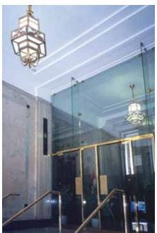
When adding any new features to meet functional requirements, adjacent character-defining elements should be conserved. A new glass wall in the Dominion Public Building in Halifax was carefully designed to complement the quality of the lobby's materials and finishes, and installed to avoid damaging the adjacent character-defining plasterwork and stone wainscoting.
