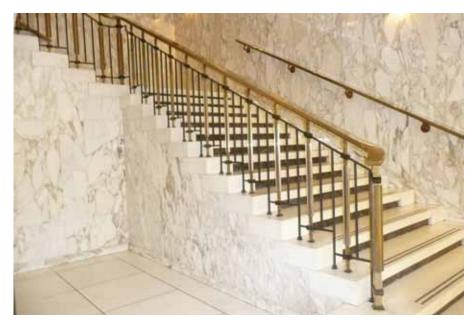
Historic guards and handrails often do not conform to current codes and safety regulations. Modifying historic balustrades in a compatible way to meet these requirements is recommended over replacement. The balustrade at the National Archives and Library in Ottawa underwent a sensitive rehabilitation to meet current requirements for spacing between balusters.
