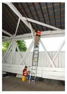
Before beginning project work, the form, materials and condition of engineering works should be documented. Heritage recording of the Powerscourt Covered Bridge, National Historic Site of Canada in Powerscourt, QC, the only surviving bridge that uses the McCallum inflexible arch construction, included detailed measurements and a photographic record.
