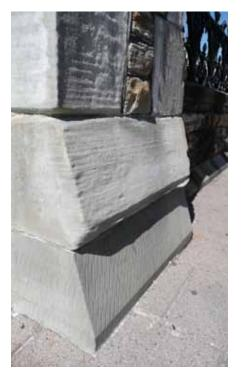
The new pieces of stone on the Wellington Wall at the Parliament Grounds in Ottawa are clearly visible on close inspection due to a different tooling technique.
