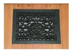
Functional elements, such as radiators and decorative grilles, can contribute to the overall heritage character of a place. Opportunities to retain these features when upgrading or replacing mechanical systems should be explored. This heating grate is one of many that were retained and repaired for use with a new heating plant when the Dawson City Telegraph office was rehabilitated into housing.
