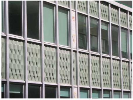
Plastic and fibreglass can be moulded into a variety of shapes to create decorative, colourful wall panels. These green moulded panels are unique and difficult to replicate if damaged. Removing intact panels from a less visible part of the building to replace broken panels in a more prominent area is one possible strategy.
