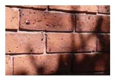
Sandblasting was once a popular method of removing paint from brick; however, it also removed the brick's outer hardened "crust" causing the brick to deteriorate.
