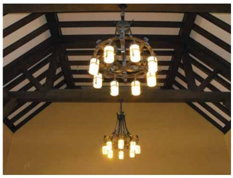
These large light fixtures in the main hall of the Jasper train station were rewired and adapted to accept compact fluorescent bulbs in order to meet sustainability and current health and safety concerns. Light fixtures of any scale can be similarly rehabilitated rather than being replaced.
