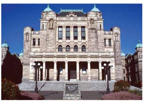
Preserving the exterior of the British Columbia Legislative Building (its rear façade shown here), including its masonry walls, steps, columns, pilasters, window surrounds, decorative details and cornices, began with documenting the material, form, jointing, tooling, bonding patterns, coatings, colour and conditions of these elements before beginning project work.
