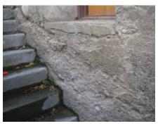
In the early 20th century, concrete was still an experimental material. The early designers and fabricators did not have full knowledge about the properties and characteristics of the concrete or its performance in the Canadian environment. Early examples of concrete construction often have inherent problems, are in poor condition and can require considerable conservation work.
