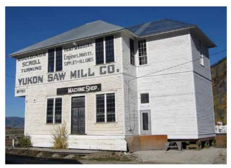
A compatible addition to the rear of the Yukon Sawmill Co. Office provides space for services. If necessary, it could be removed without affecting the building's historic fabric. One window opening and the surrounding wall framing were altered to provide space for a connecting door.
