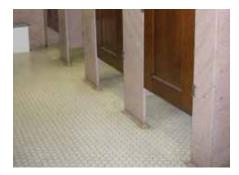
Mass-produced elements, such as ceramic tiles, are frequently used in buildings. Finding matching replacements for repair work can be almost impossible. If tile needs to be removed from one area, it is good conservation practice to save nd stockpile it for later use elsewhere in the building. These tiles from the washrooms in Union Station in Toronto were removed from one set of washrooms in order to provide a stockpile of tiles to use in the repair of the remainder of the washrooms.
