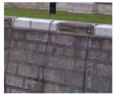
Masonry: In this rehabilitation project of the Rideau Canal, some of the original limestone blocks remained in good condition. Others, which were too deteriorated to repair, were replaced in kind with new limestone blocks.
