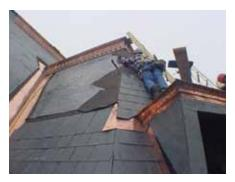
The Rehabilitation of the Truro Post Office, in Truro, NS included restoring its distinctive slate roof. In Rehabilitation, the replacement of missing historic features with a replica based on physical and documentary evidence, as in this project, is acceptable, as is a new design that is compatible with the heritage value of the historic place.
