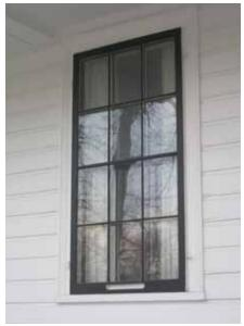
The type of glass and its division into multiple lights often defines the character of windows in historic buildings. The reflective quality of double-glazing from double sashes or storm windows is different than that of modern insulated glass. Inspections should be undertaken regularly to ensure that glazing putty is in good condition.
