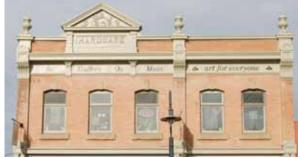
The two remaining decorative sheet metal urns at the top of the façade of the M & J Hardware Building in Lacombe, AB were determined to be beyond repair due to weathering over time. A third sheet metal urn (centre) was missing. The existing deteriorated elements and photographic documentation were used to replicate these elements. The M & J Hardware Building is an example where missing features from the restoration period have been re-instated based on physical and documentary evidence.
