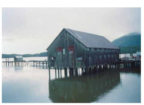
It is important to identify the cause of any damage to a wooden building element before beginning a Preservation treatment. For the former machine shop of the North Pacific Cannery in Port Edward BC, exposure to marine conditions caused the exterior wood cladding to deteriorate.
