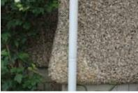
Certain stucco treatments, such as pebble-dash stucco, are difficult to replicate. Applying glass or rocky aggregate to the wet stucco is an art that is all but lost. Pebbles imported from Scotland for the Dr. Woods House in Leduc, AB are virtually impossible to replicate. The repairs resulted in a sound exterior envelope, but are clearly distinguishable from the original.
