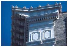
One of the primary causes of deterioration of glazed architectural terra cotta, like that shown on the Confederation Life Building in Winnipeg is water. Water-related damage to the glazed units, mortar, metal anchors or masonry backfill can be repaired only after eliminating the sources of that water. In order to ensure that the actual root problem is being solved, investigation work would need to be completed prior to any repairs in order to identify that source.
