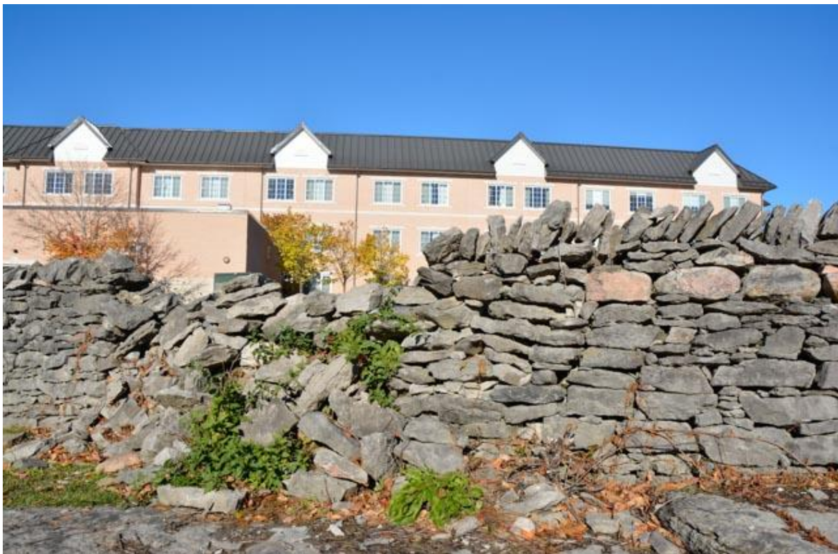
Figure 9 Wall at Mid-West end collapsed
