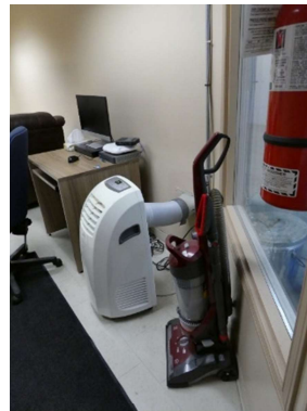
Floor mounted A/C unit vented to garage bay
