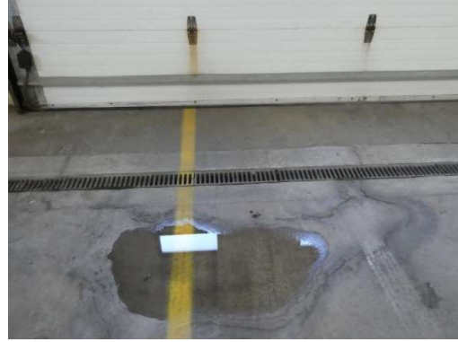
Original slit drains and existing ponding
