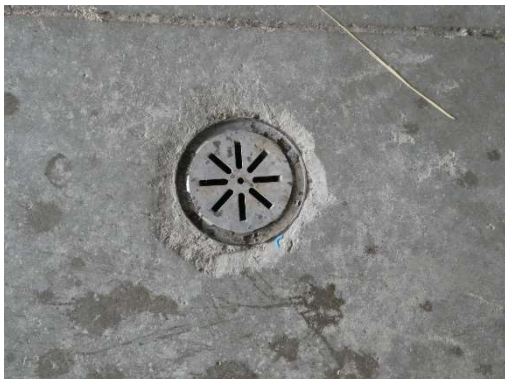
Single small round garage floor drain
