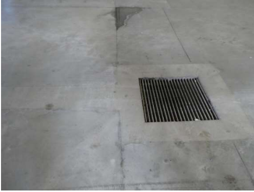
Additional square box drain to improve floor drainage
