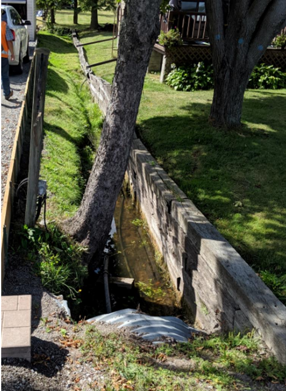
Image 6: (Picture of watercourse at inlet to 800 mm CSP pipe crossing Long Beach Road)
