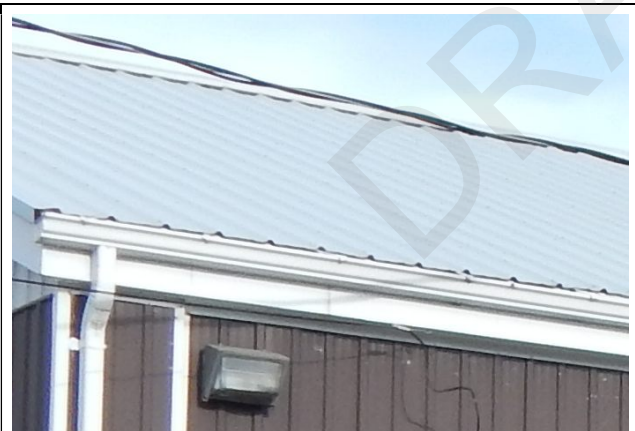
Overview of main roof
