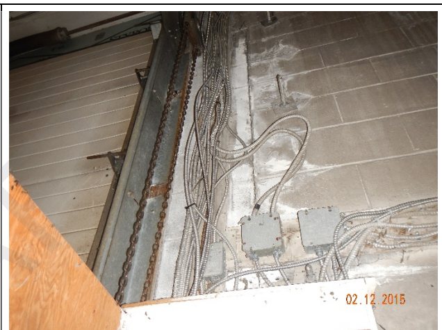
Interior concrete block wall
