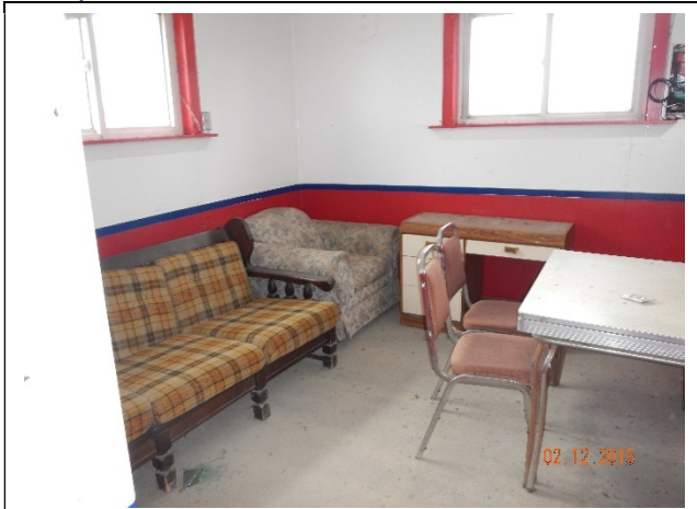
View of slab on grade floor
