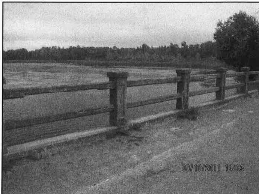
Photo 8: Localized spalls on curb and railing posts
