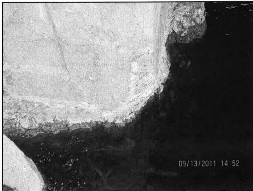
Photo 4: Severe erosion of north abutment footing
