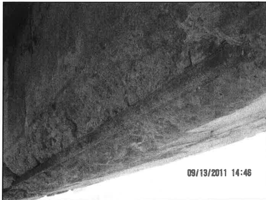
Photo 6: Spall and delamination on exterior west beam
