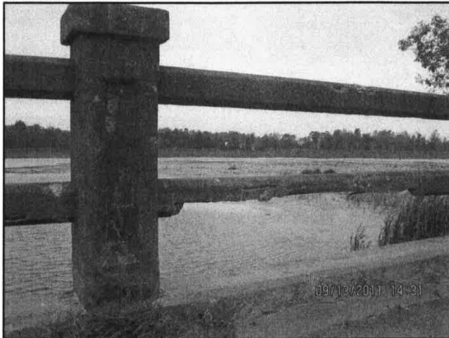
Photo 5: Spalls and section loss on west railing
