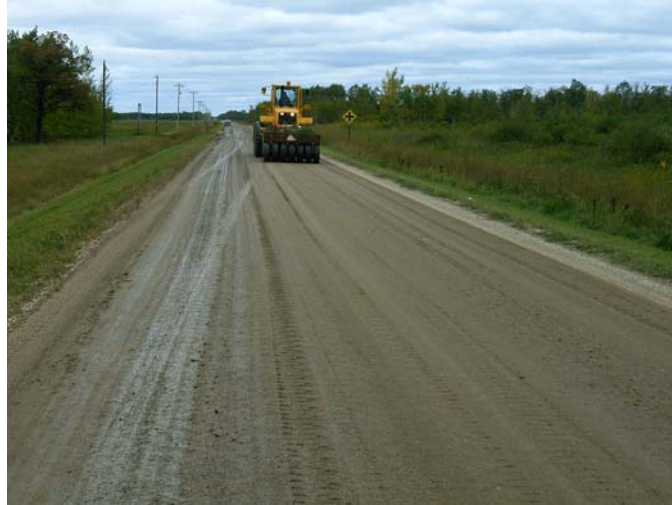
Figure 4 Rolling treated aggregate surface, Pennington 72.
