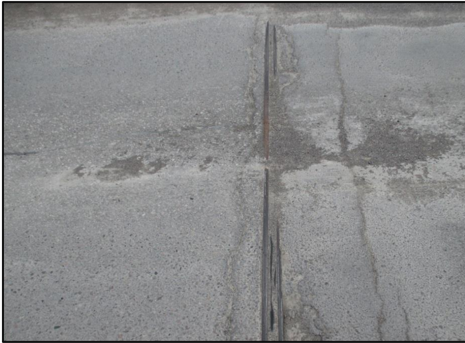
Photo 3: Jammed joints (typical of both ends)
