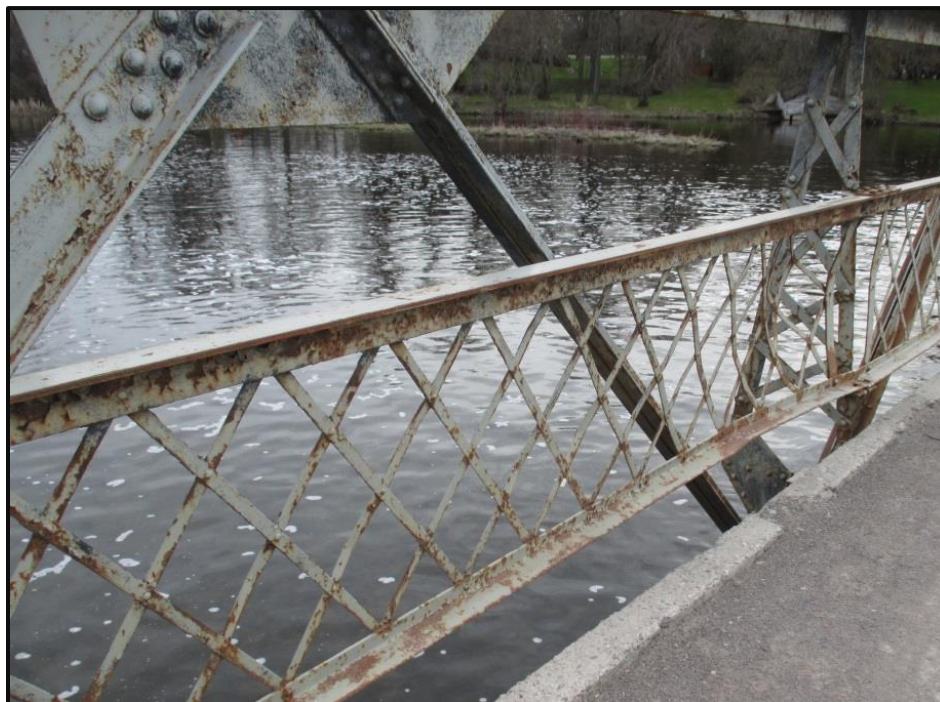
Photo 5: Deformed railing
