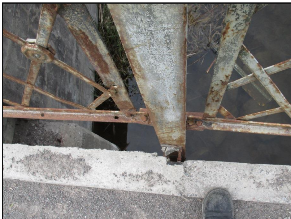
Photo 6: Broken post at southeast
