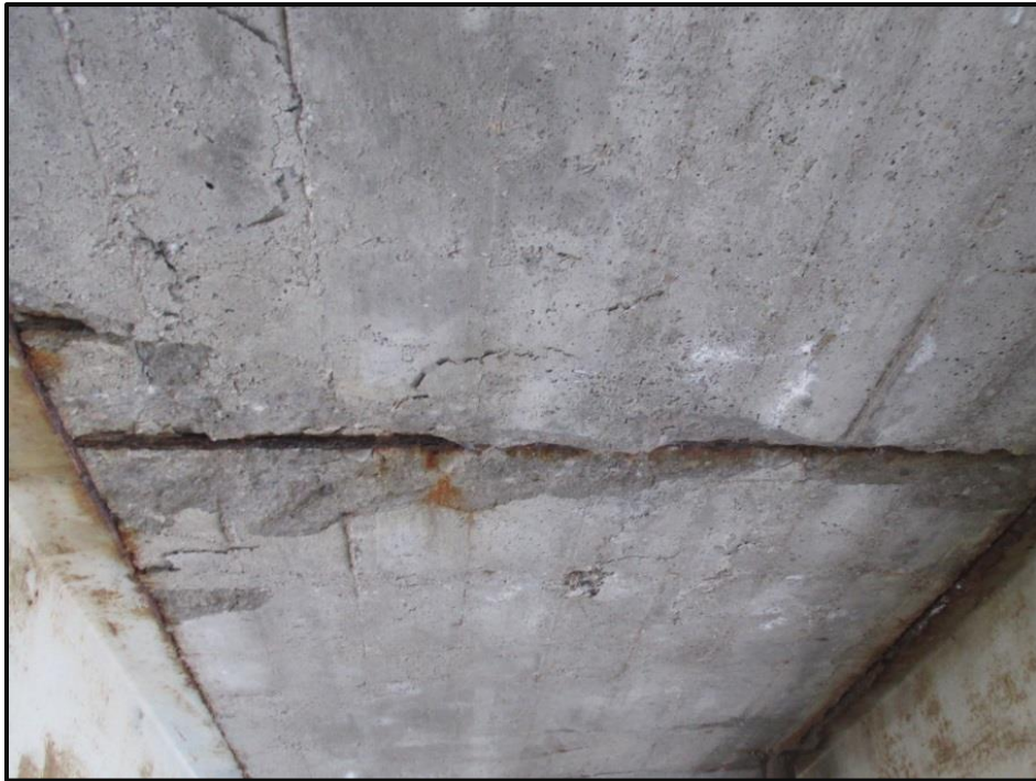
Photo 7: Severe spall at soffit (typical of soffit)
