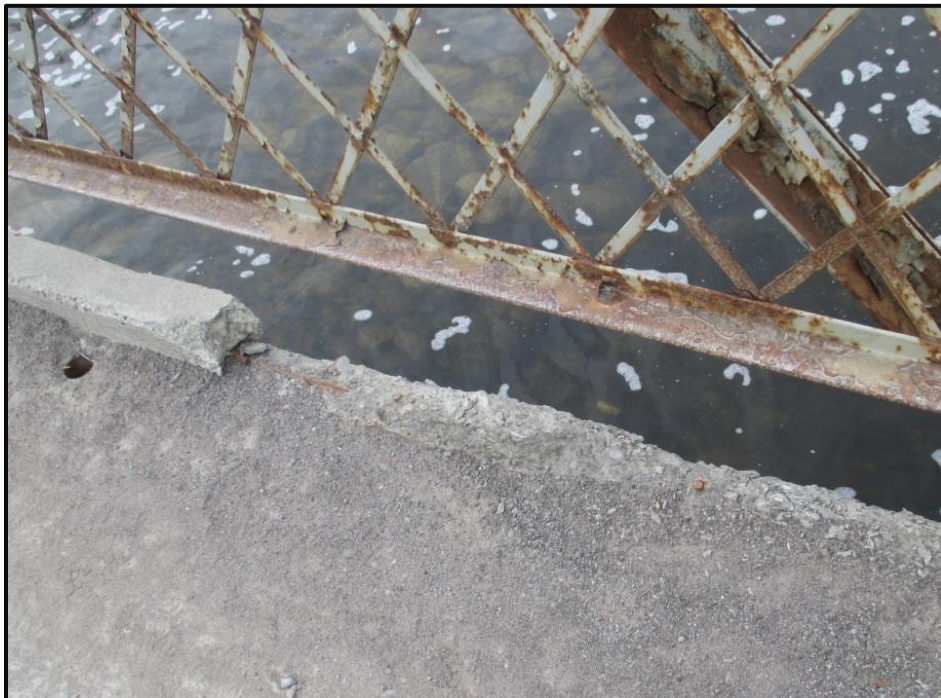
Photo 4: Typical spalling at curb
