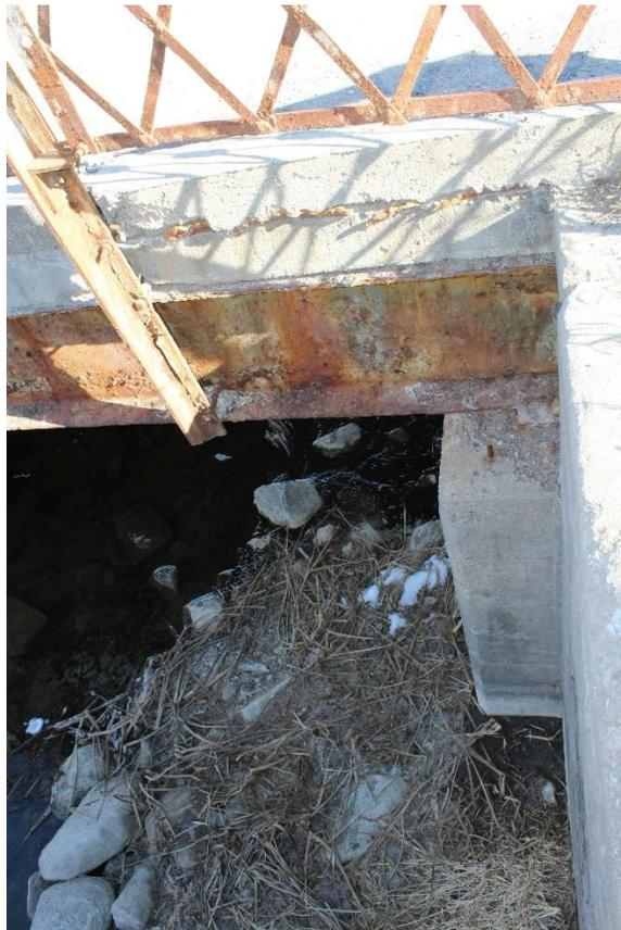
Plate 22: View of concrete abutment and bearing seat on the east abutment, looking north from the southeast quadrant of the bridge.
