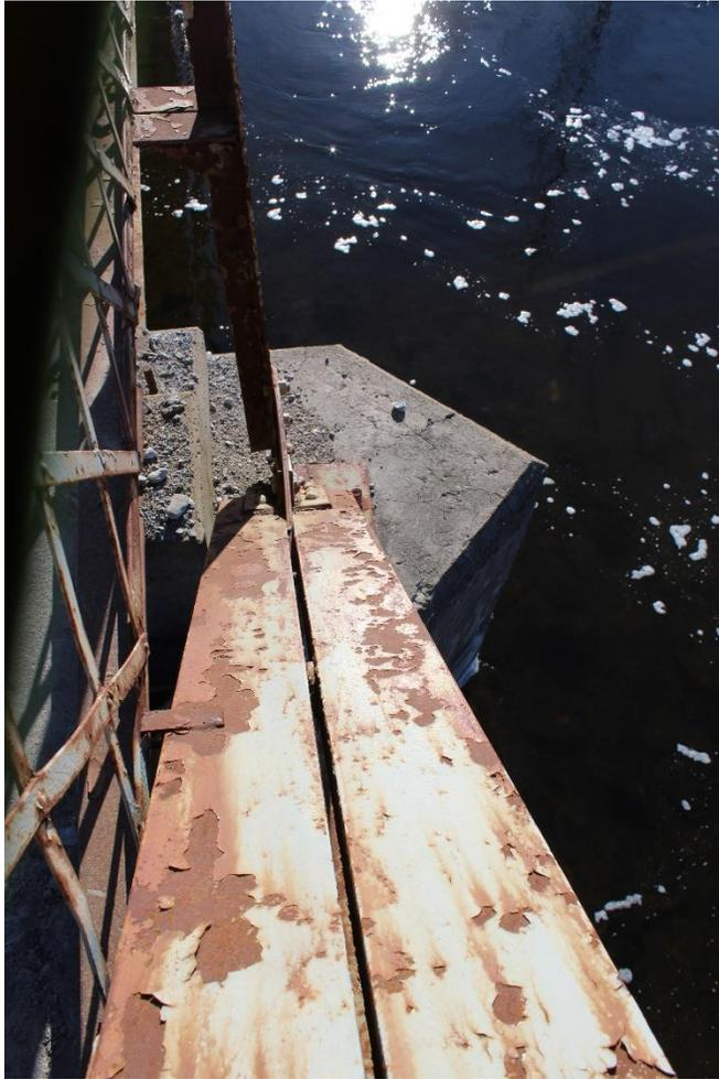
Plate 13: View of top of the western pier with pointed upstream face.
