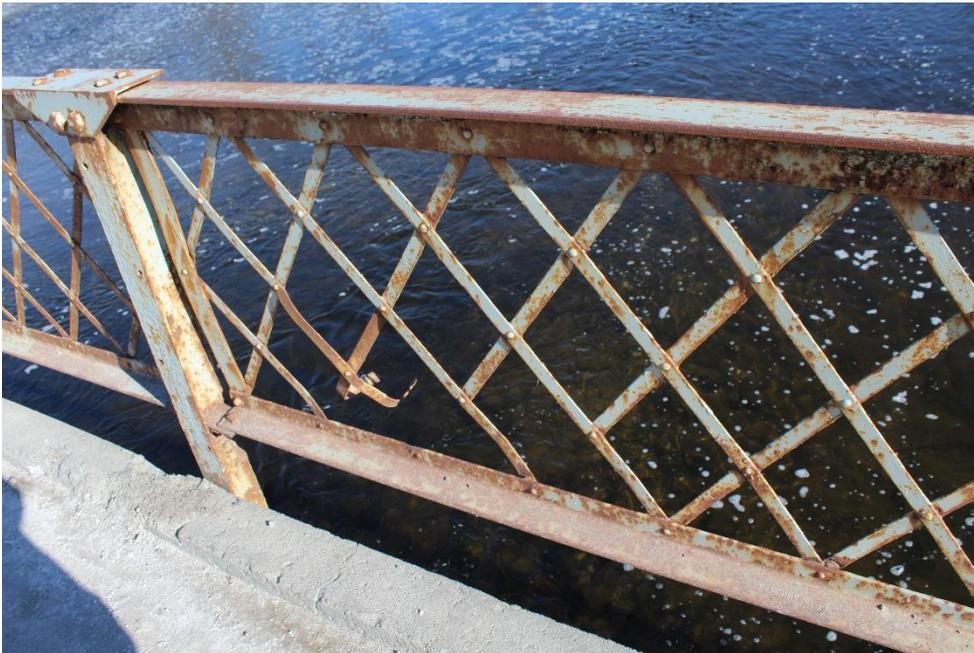
Plate 17: View of damage to steel lattice barrier.
