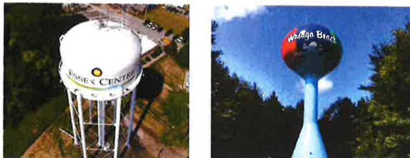
Figure 1: Photo of the recoated and rehabilitated Essex Water Tower and Wasaga Beach Water Tower.
