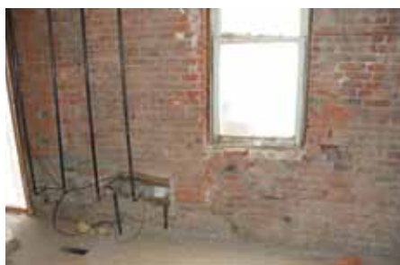
Left: Interior of west (rear) wall of north retail bay, showing as-found condition of load-bearing masonry after removal of the lath and plaster interior finishes for inspection purposes. Uncontrolled runoff from the roof had saturated the wall, washed out the mortar, and caused localized collapse around the window opening.
