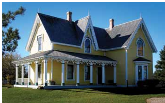
Based on documentary evidence, including an 1880 engraving, the original fenestration of the Biddeford Parsonage Museum in P.E.I. was restored and roof finials replaced.
