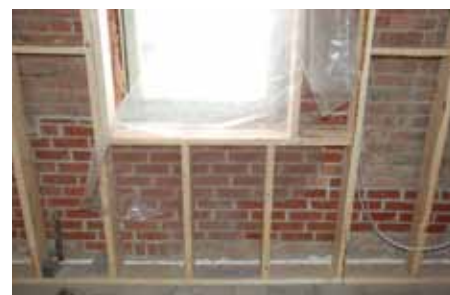
Left: Interior of west (rear) wall of north retail bay, showing as-found condition of load-bearing masonry after removal of the lath and plaster interior finishes for inspection purposes. Uncontrolled runoff from the roof had saturated the wall, washed out the mortar, and caused localized collapse around the window opening.
