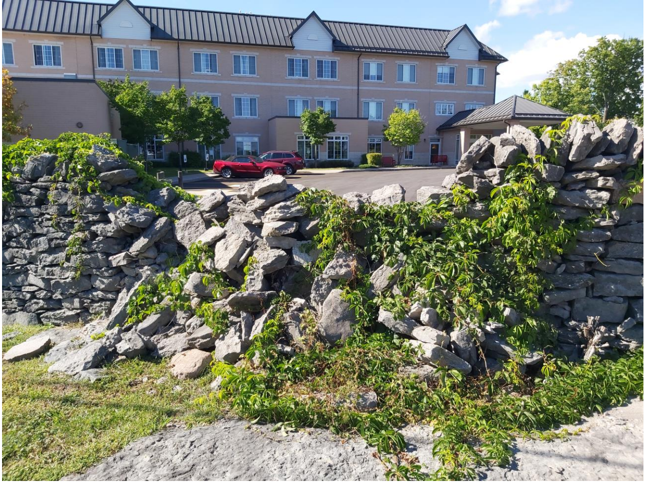
Section of wall requiring repairs
