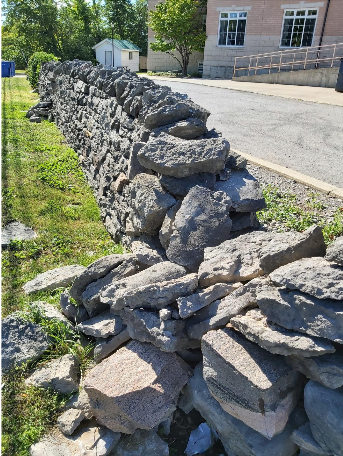
Evidence of double wall construction
