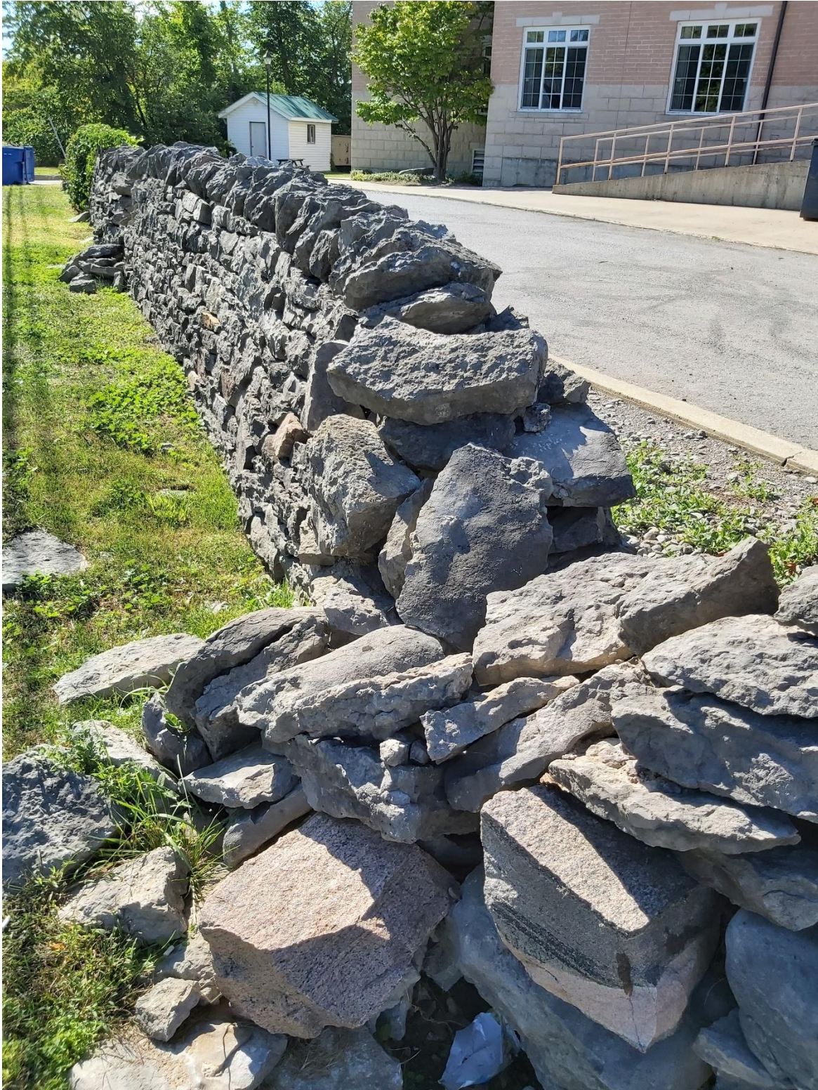
Evidence of double wall construction
