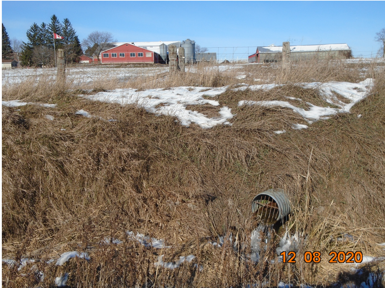
Tile drainage out letting to the north side road ditch on County Rd.# 36 east of Snug Harbour Rd.
