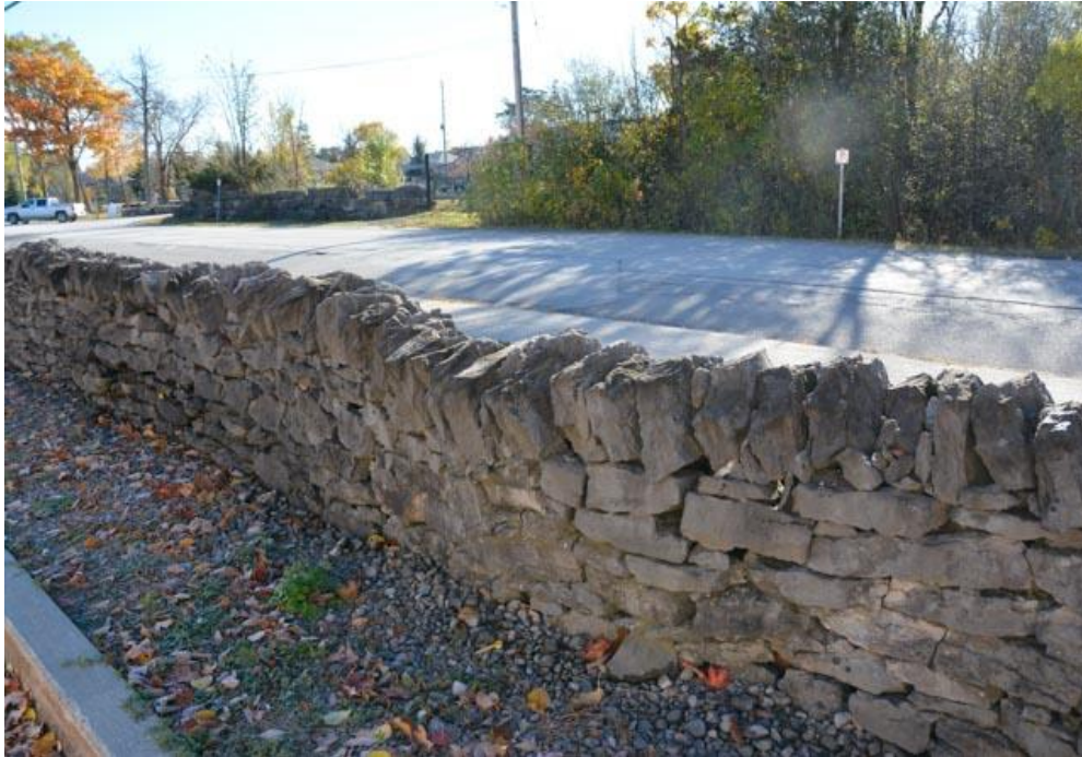
Figure 8 Wall at the West end of property “leaning”
