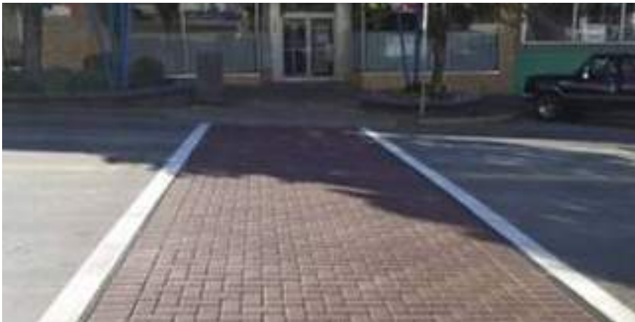
Asphalt cross walks are highlighted with a complimentary stamped pattern and colour, and are further defined with a bright white painted band.
