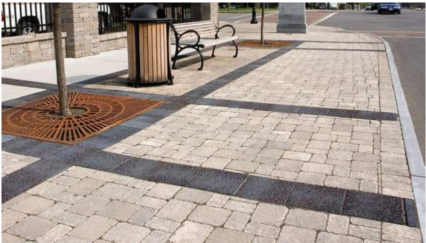
Concept B ‘Ribbon Pattern’: Dark granite like pavement banding separates the sidewalk and furnishing zones.
