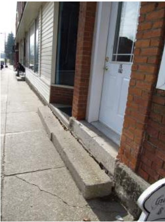
Business entrances not level with sidewalk- requires stairs up into buildings. Ramps without handrails provide obvious challenges and add to obstruction on street.
