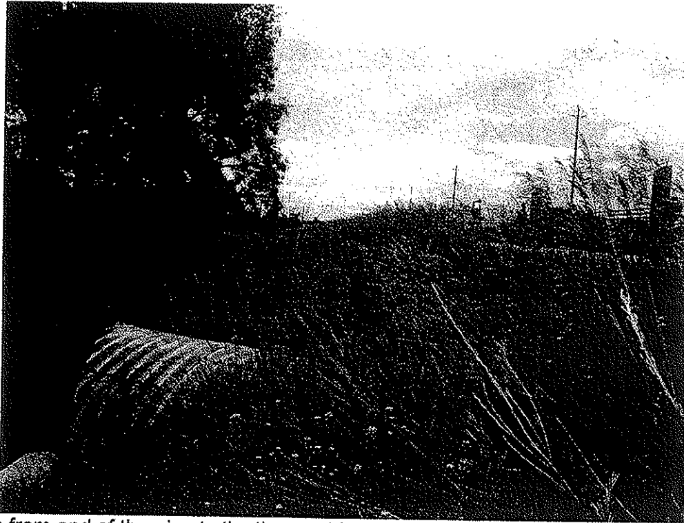
5.0 metres from end of the pipe to the three cable guide rail.
