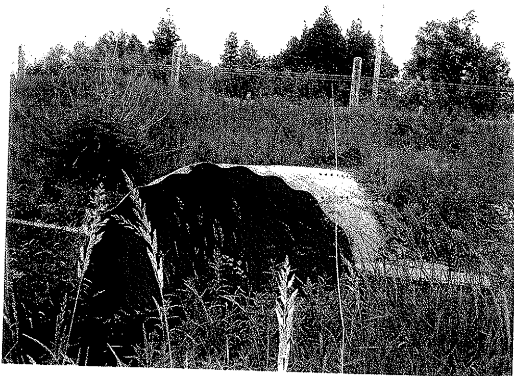
1.8 x 3.0 CSPA with Concrete wingwalls, 0.9 km north of Hwy 7 on the east side of CKL 36
