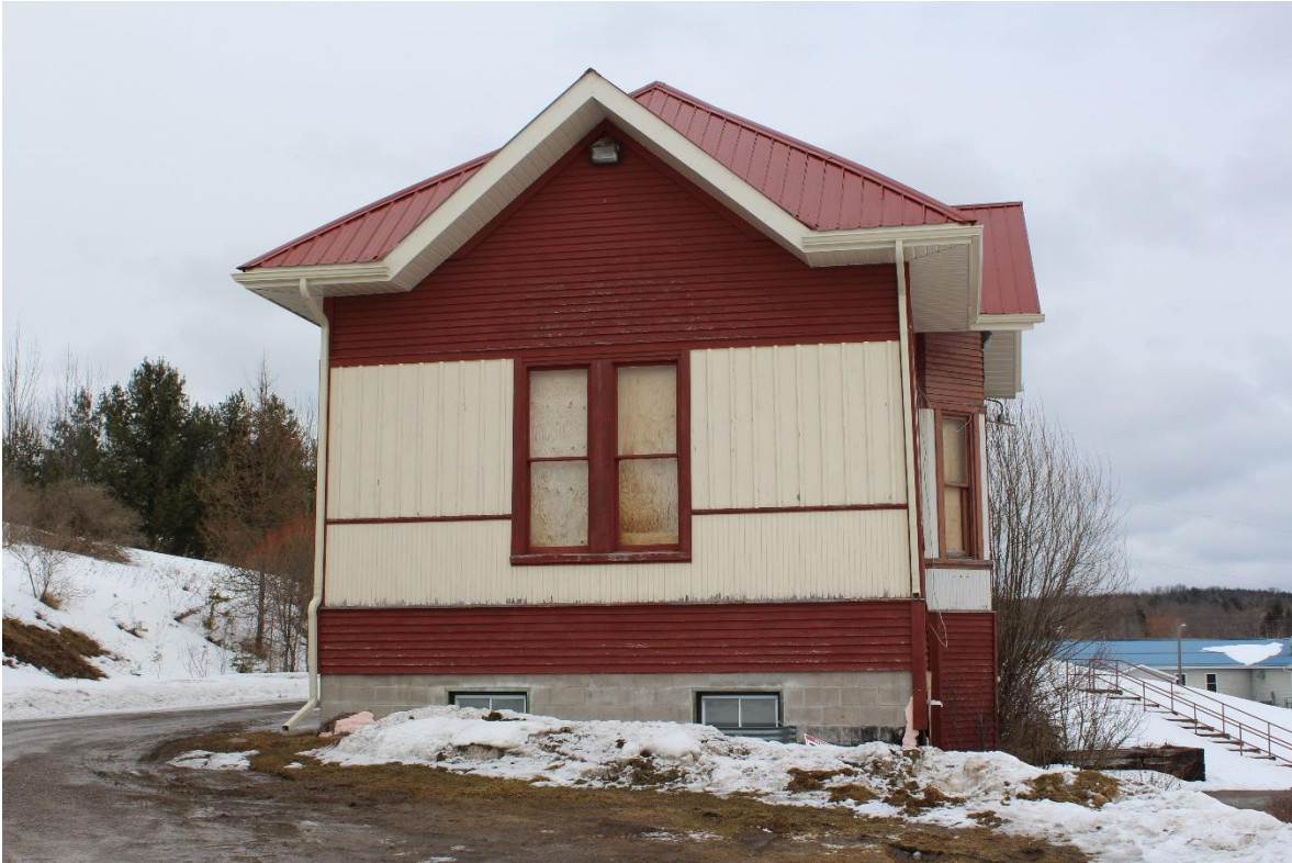
West elevation, March 2022
