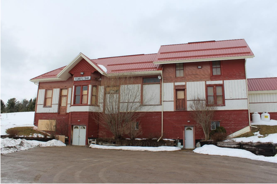
South elevation, March 2022
