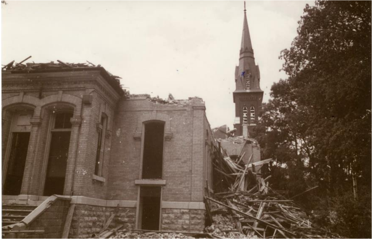
Demolition of the convent (1977), Kawartha Lakes Public Library
