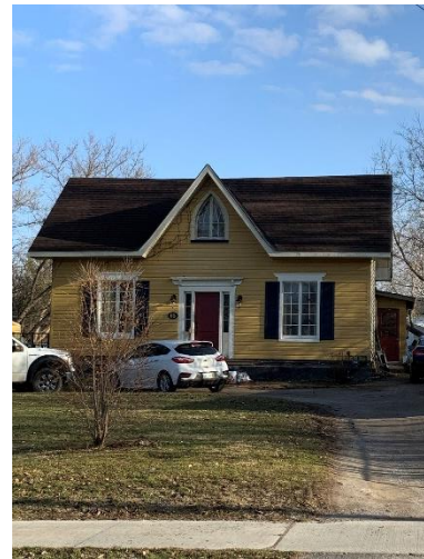
65 Glenelg Street East
