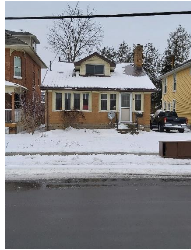
4 Glenelg Street East
