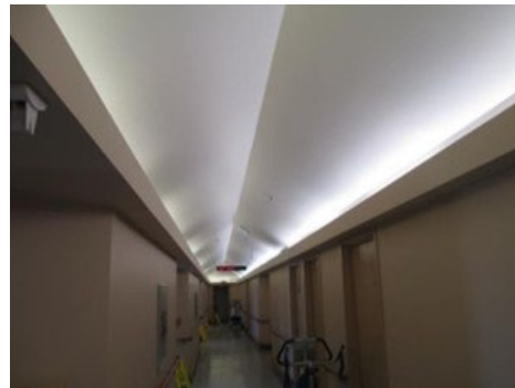
Figure 14 – Interior Door & Wall Finish
