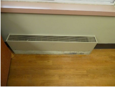
Figure 23- Perimeter Heating
