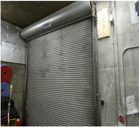
Figure 10 - Rolling steel door Loading Dock
