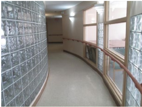
Figure 13 – Floor Finish Home Area Corridor
