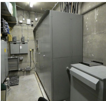
Figure 27 – Main Switchgear
