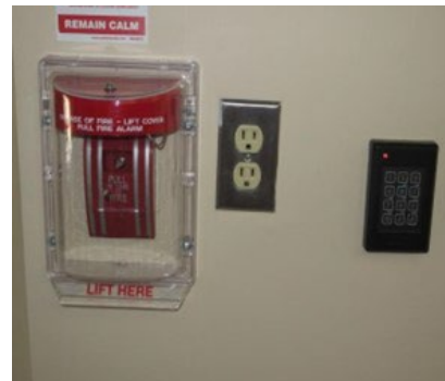
Figure 32 – Pull Station
