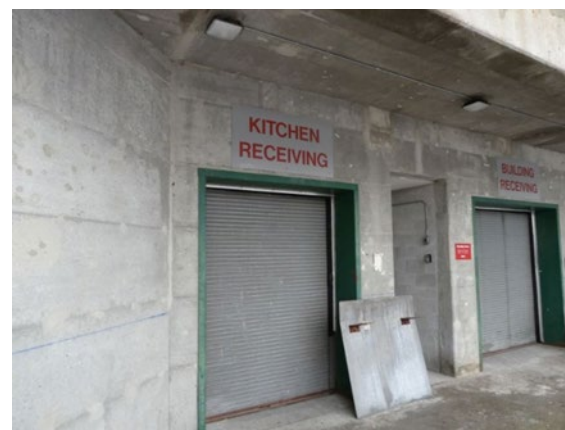
Figure 9- Exterior steel rolling doors
