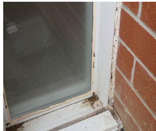
Figure 8 - Exterior Window Sealants
