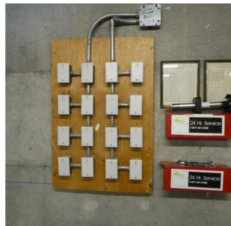
Figure 2 – Foundation Wall – Fire Pump Room Basement Level
