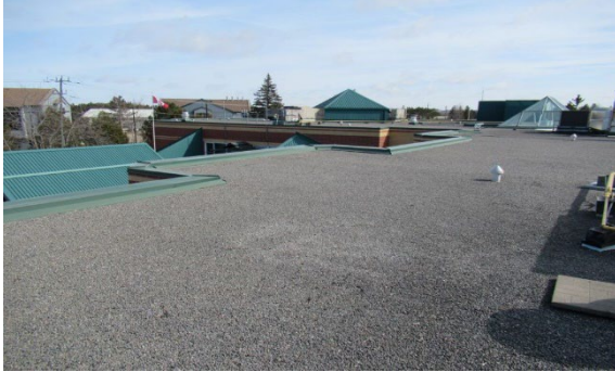
Figure -12 Roof Covering
