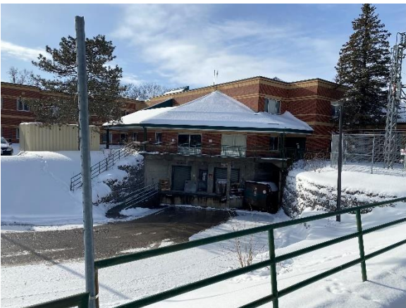
Receiving Area - Exterior
