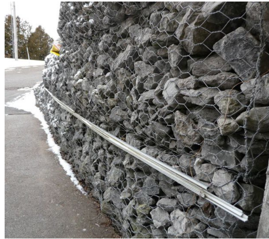
Figure 39 – Stone retaining wall wire meshing Loading Dock
