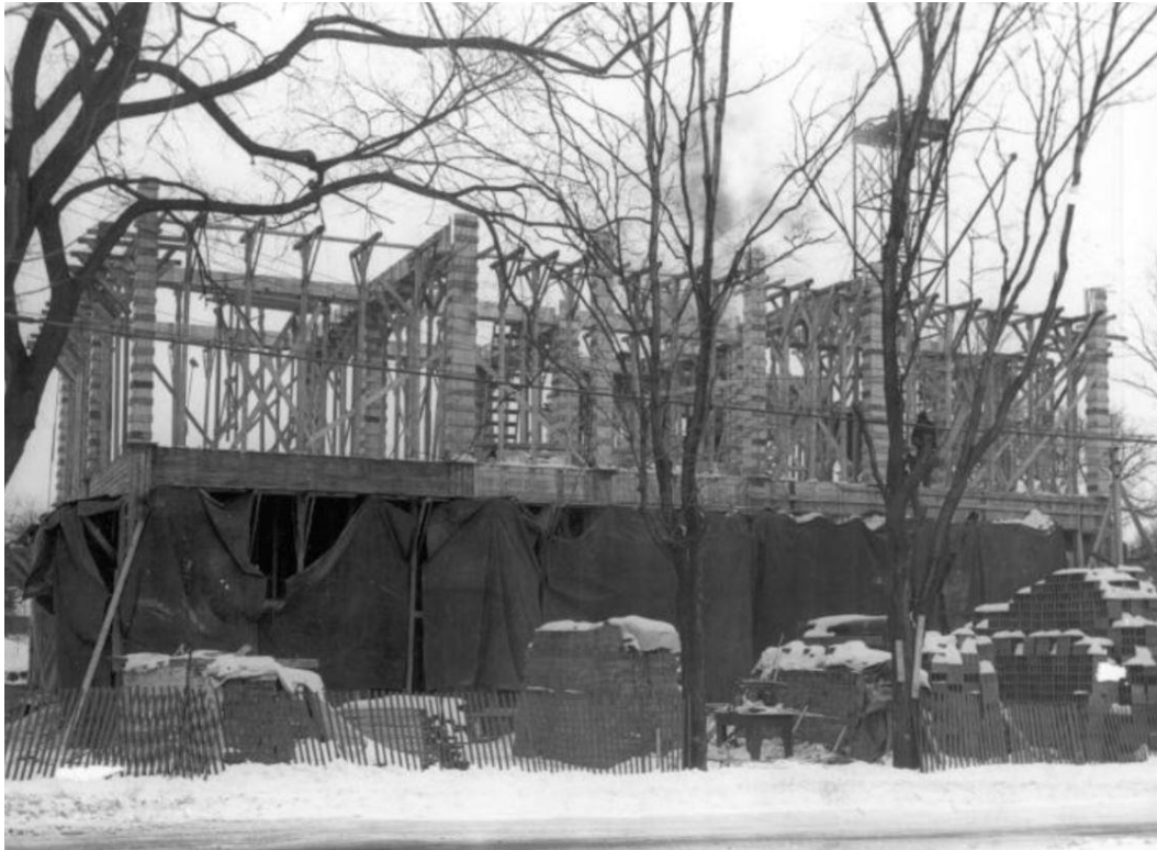
91 William Street North under construction, c.1949 (Bell Canada Archives)
