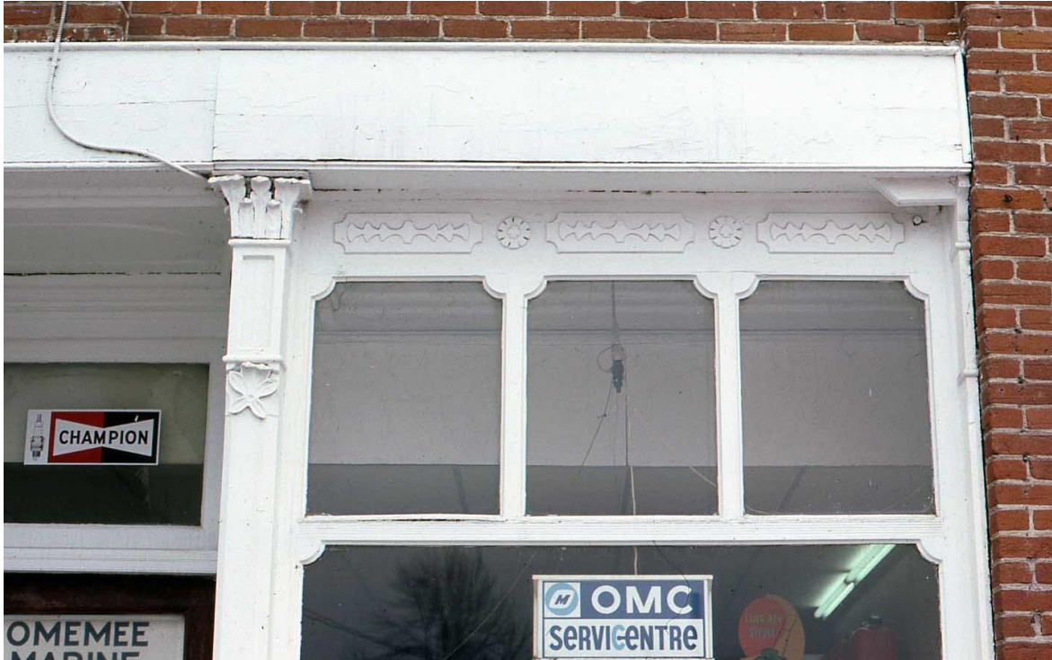
Cast iron storefront details, c. 1977
