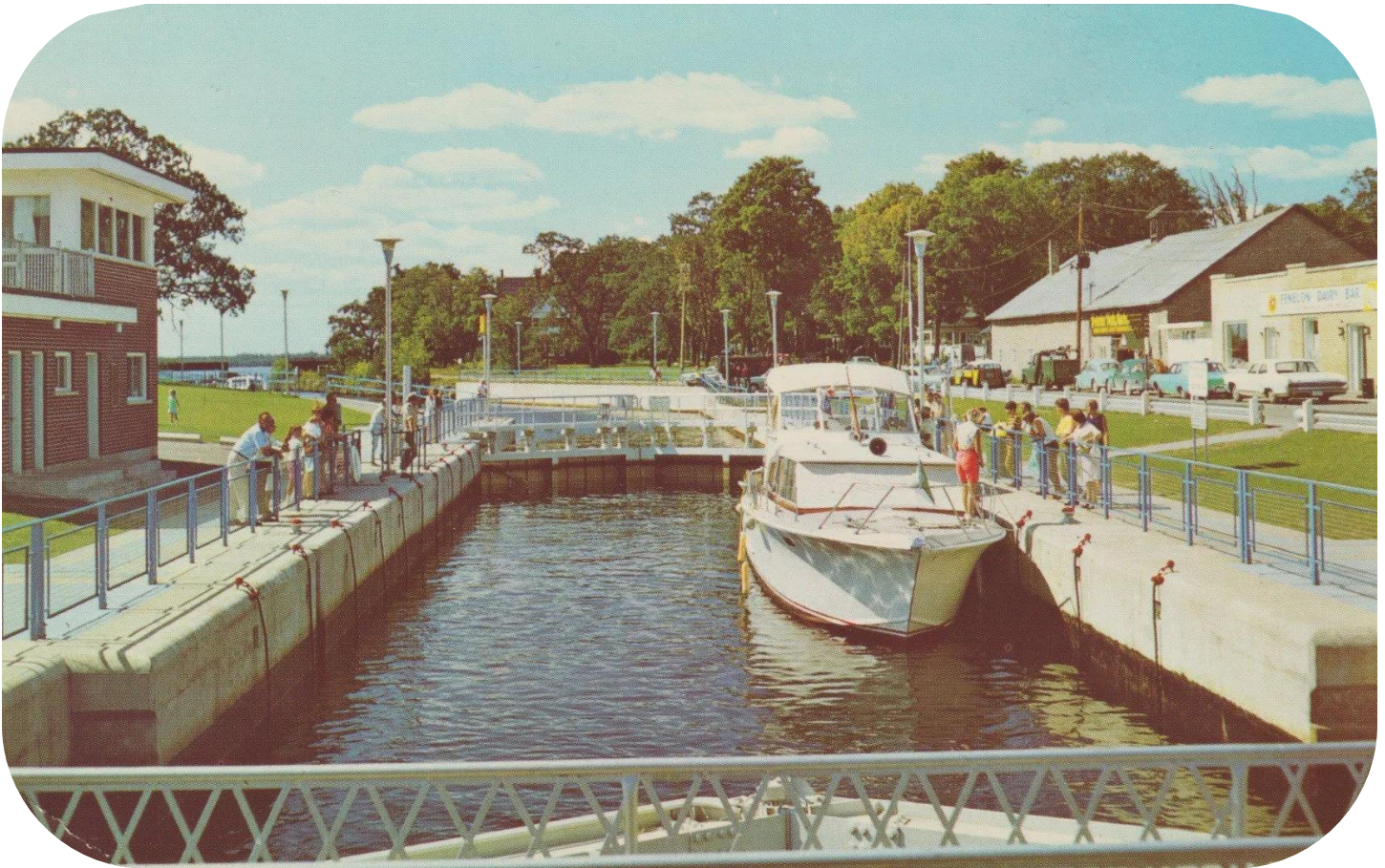
Boat in the Fenelon Falls Lock, 1975
