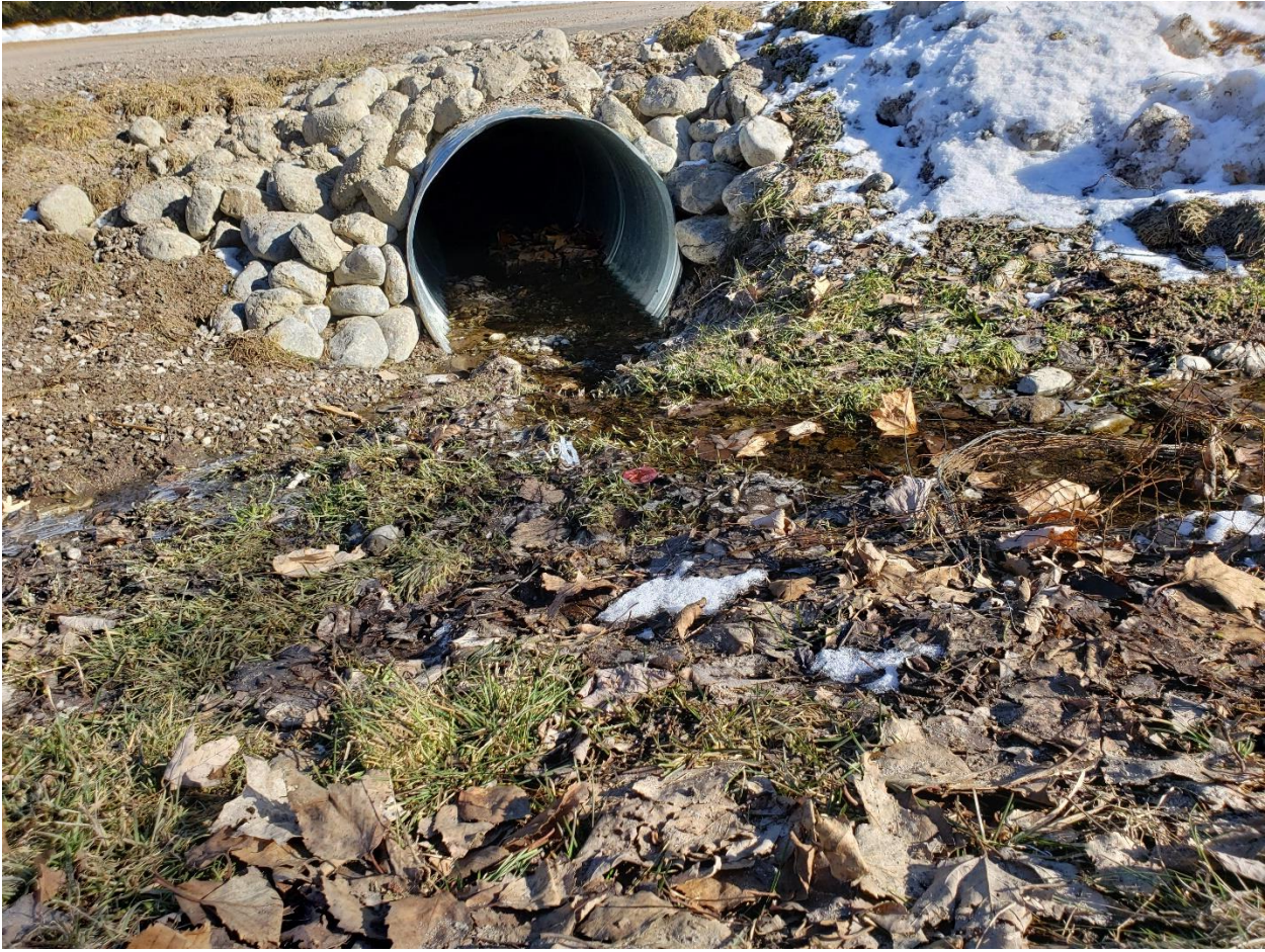
Cameron Dr. cross culvert inlet
