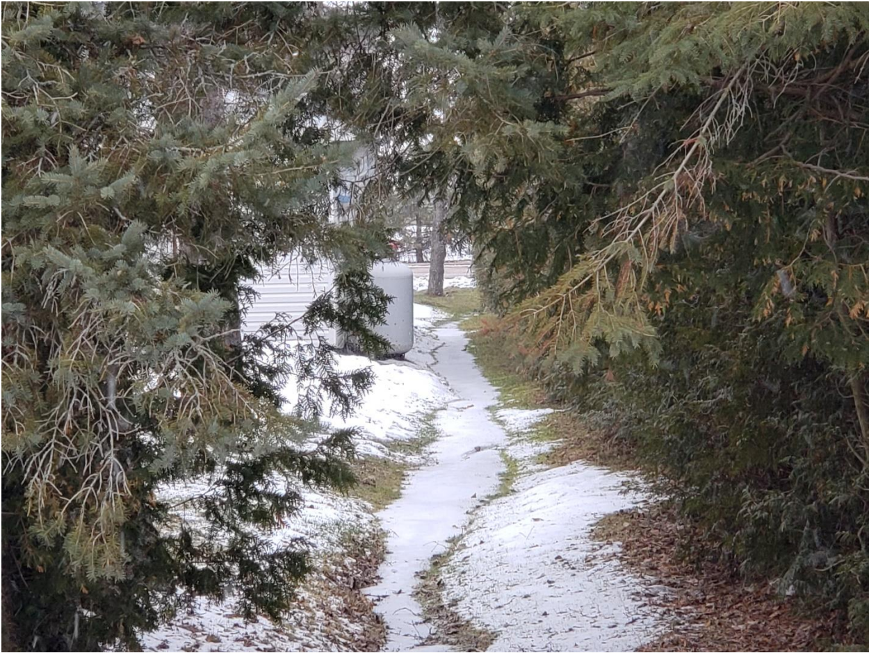
Another view of swale on 149 Fenelon Dr.
