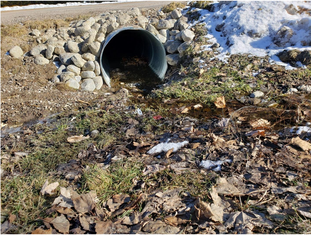
Cameron Dr. cross culvert inlet
