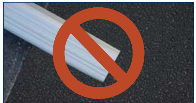
Avoid directing downspouts across paved surfaces.
