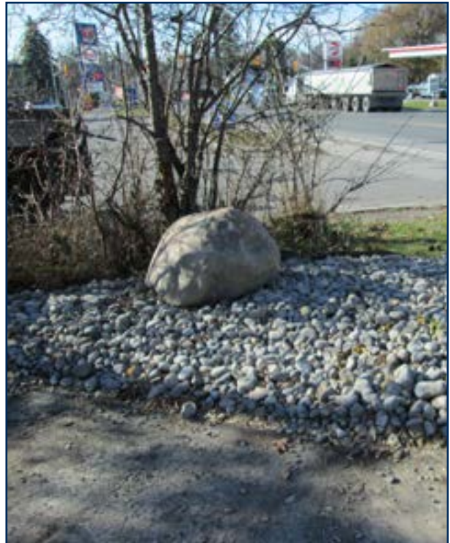
A soakaway pit at the end of the trench
