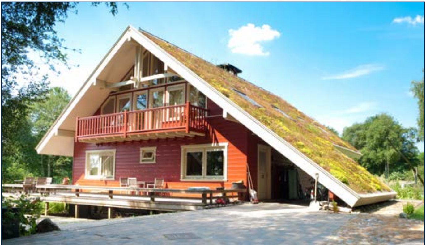
Green roof benefits: reduces runoff and urban heat island effect, adds to urban ecology and has longer lasting construction.
