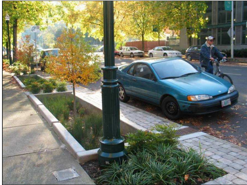
Figure 14 – Extended tree pit bioretention designed to capture street runoff (Source: City of Portland Bureau of Environmental Services)
