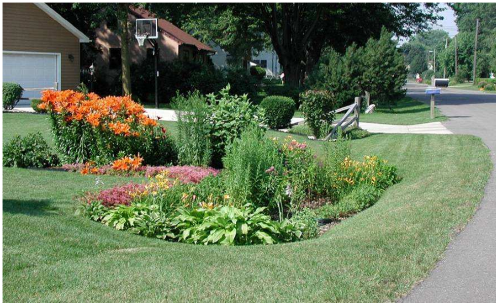
Figure 20 – Residential rain garden in Maplewood, MN (Source: City of Maplewood, MN)
