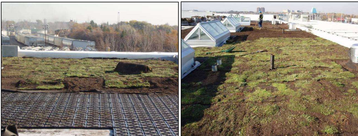
Figure 7 – GO Transit bus facility extensive green roof installation with pre-grown mats, Mississauga, ON (Source: CVC)
