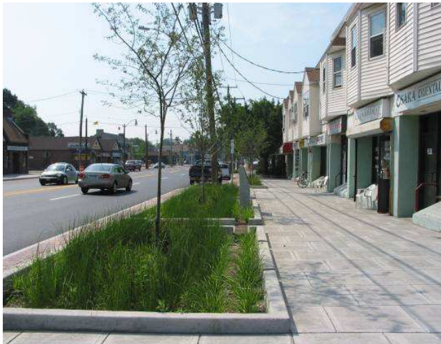
Figure 2. Urban stormwater planters are incorporated into a constrained urban streetscape in Bridgeport, CT with ornamental grasses and trees. (Source Talledega Design Group)
