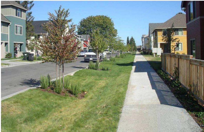
Figure 28 – Manicured shallow grass swale combined with areas of herbaceous plantings and trees between the curb and sidewalk in Seattle, WA (Source: SVR Design Company)
