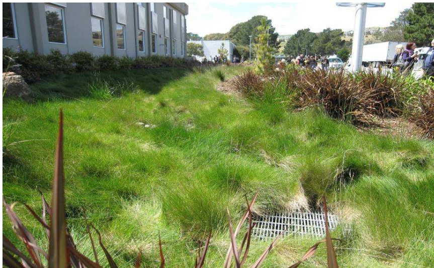
Figure 29 – A no mow grass swale in Brisbane, CA (Source: CVC)
