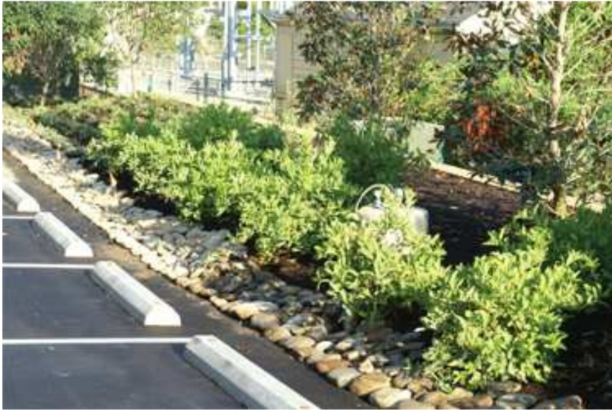
Figure 25 – Filter strip planted with shrubs and herbaceous plants treating a parking lot with no curbs in the Hill Center project in Green Hills, TN (Source: Hawkins Partners, Inc)
