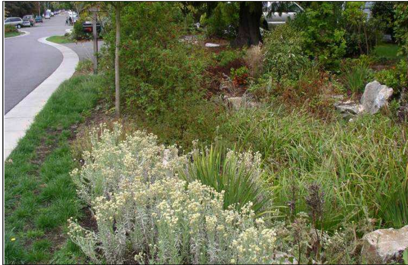
Figure 31 – Dry swale constructed as part of the Seattle Public Utilities Street Edge Alternative program. (Source: Center for Watershed Protection)
