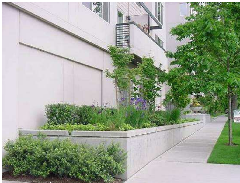
Figure 18 –Lined stormwater planter accepting runoff from residential building rooftop, Portland, OR (Source: Portland Bureau of Environmental Services)
