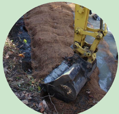
Coir fabric installation
