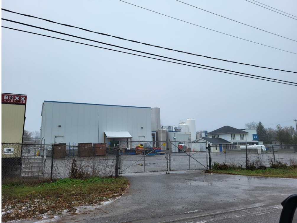
Truck entrance and facilities Direction: east from Head Street
