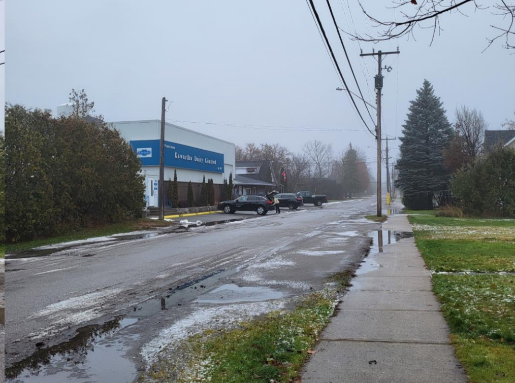
Prince Street West Direction: northeast from Head Street and Prince Street West
