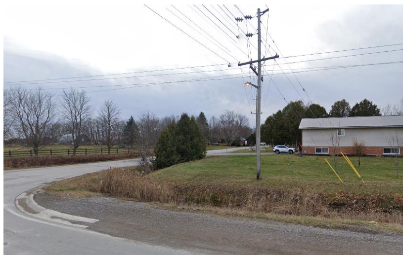
Figure 1: Picture of private light, facing west on Highway 7 – Google, Dec. 2022
