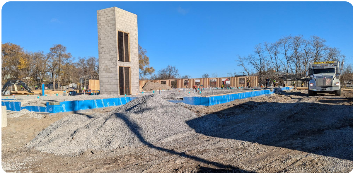
Construction site of 70 Murray Street, Fenelon Falls
