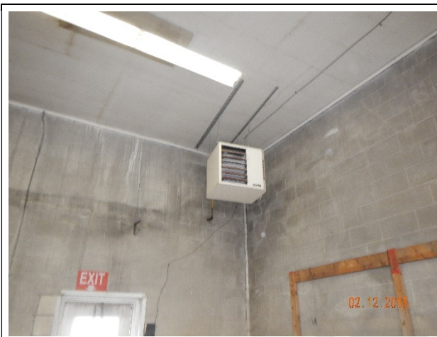
Interior concrete block walls
