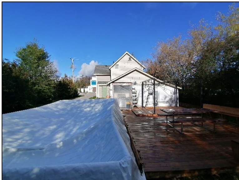
Figure 49: Rear elevation (MHBC, November 2021).
