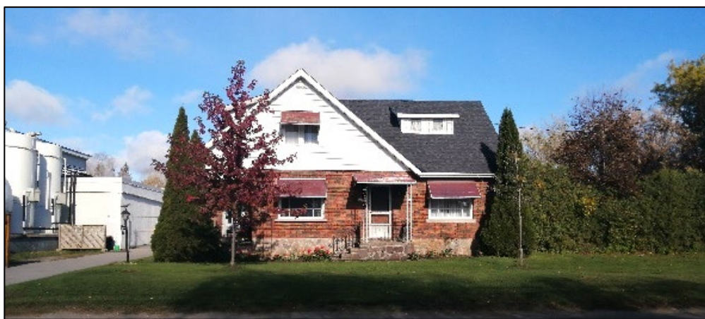
Figure 31: Street-facing (south) elevation of the building at 83 Prince Street (MHBC, November 2021).
