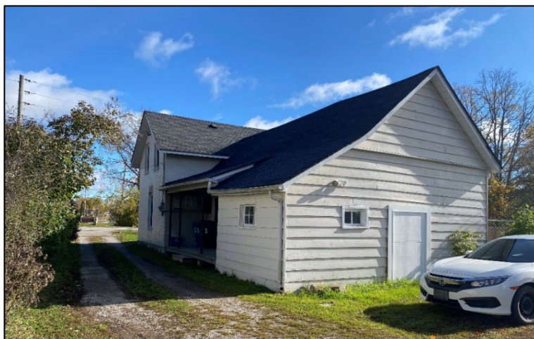
Figure 22: North elevation, facing east (MHBC, November 2021).
