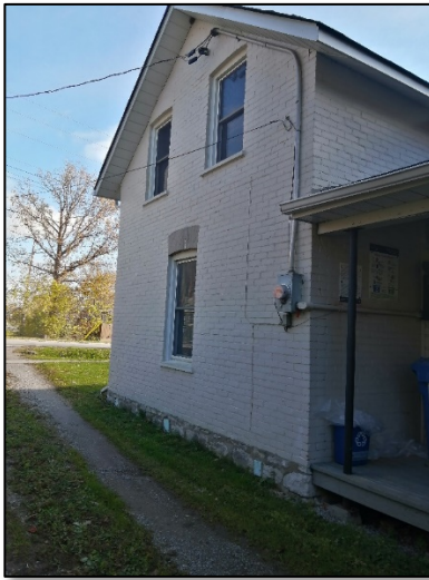
Figure 23: Original portion of north elevation (MHBC, November 2021).
