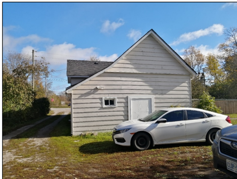
Figure 24: Rear elevation facing east (MHBC, November 2021).
