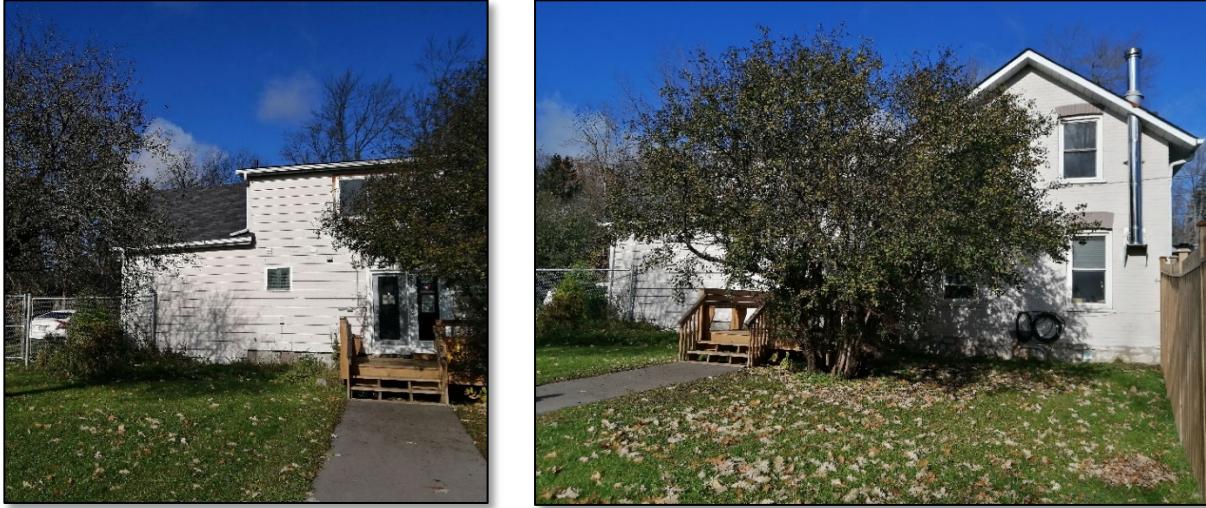
Figures 25 & 26: South Elevation (MHBC, November 2021).
