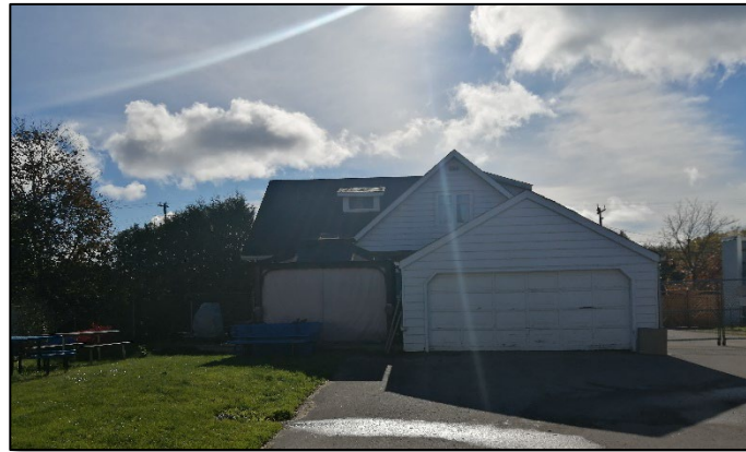
Figure 34: Rear elevation of the building (MHBC, November 2021).
