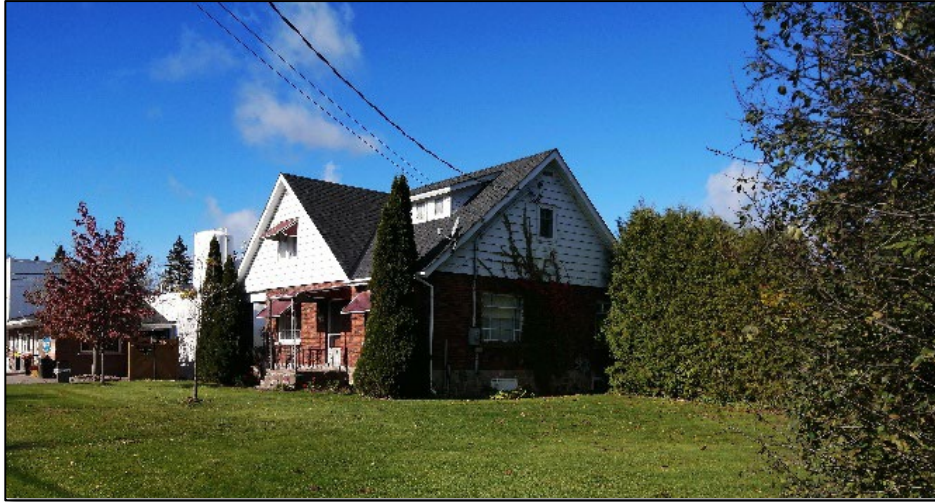
Figure 32: The side (east) elevation, facing northwest (MHBC, November 2021).
