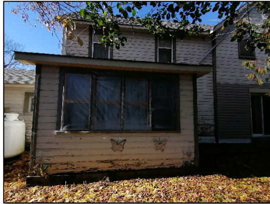
Figure 44: Central addition on east elevation (MHBC, November 2021).
