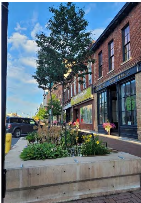
Kent Street silva cell installation to help with urban runoff and reduce the heat island effect.
